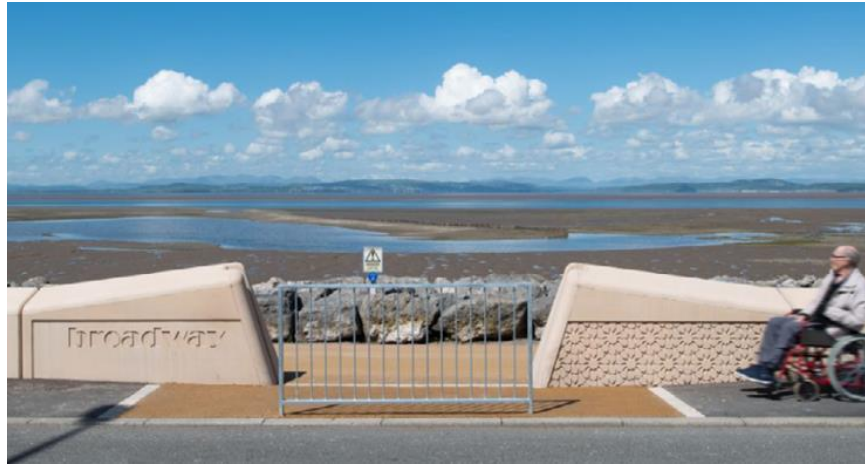
Promenade Seawall in Morecambe, UK ©Atkins
