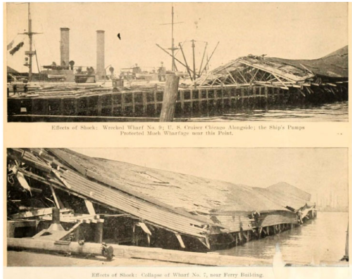
Figure 3-4. Damaged Piers after the 1906 Earthquake
