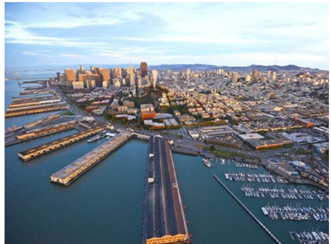
Looking south toward several of the Port's overwater marine structures.
