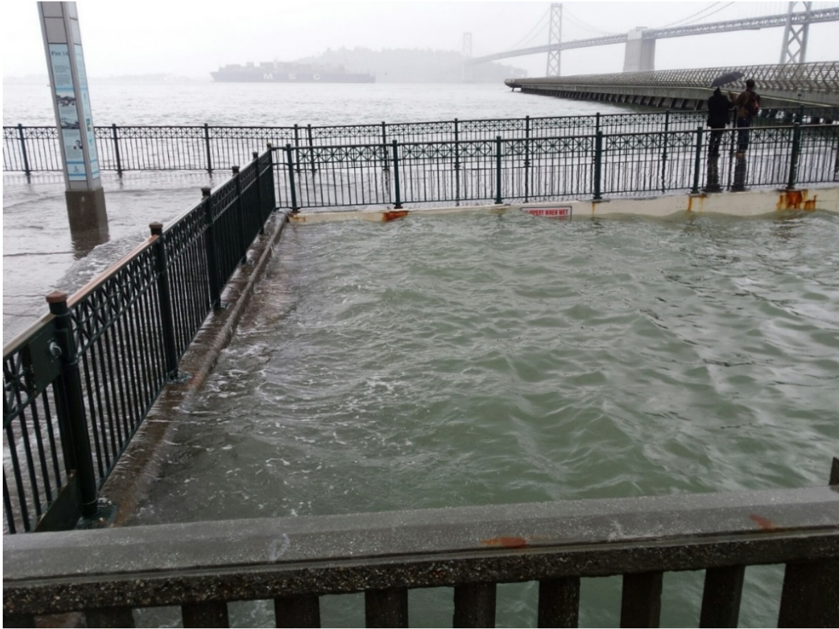
Figure 5. San Francisco Bay waters spilling onto the walkway immediately southeast of the Agricultural building (Photo by George Fong)
