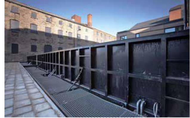
Deployable Flood Barrier
