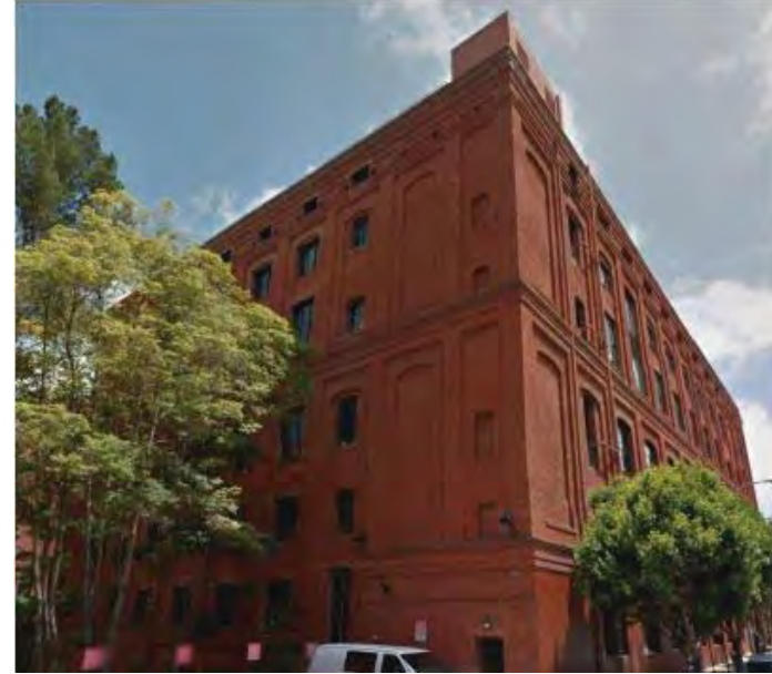
BUILDING EXAMPLE WITHIN DISTRICT Ice House, 1150 Sansome St.
