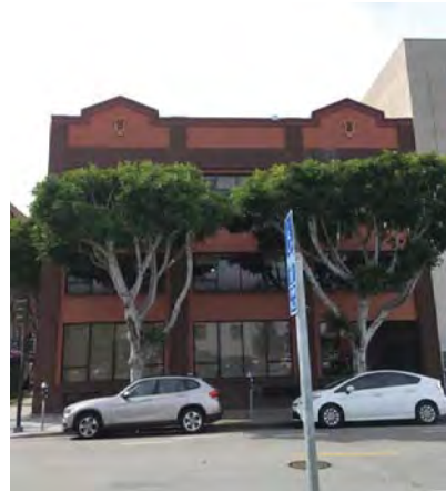
FRAME AND INFILL WITHIN DISTRICT 100-120 Broadway
