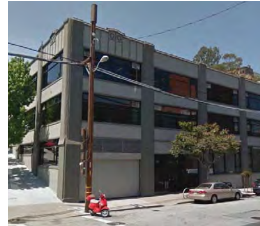
FRAME AND INFILL WITHIN DISTRICT 1005 Sansome St.
