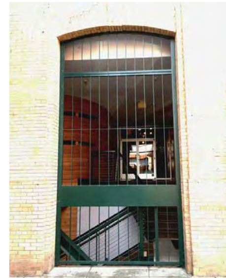
TRANSPARENCY/GATES WITHIN DISTRICT 55 Union St.
