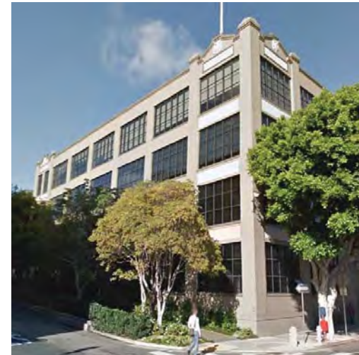
FRAME AND INFILL WITHIN DISTRICT 901 Battery St.
