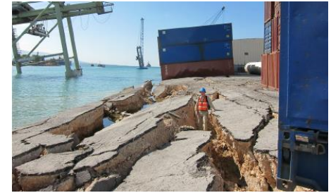
Liquefaction induced lateral spreading at Port de Port-au-Prince
