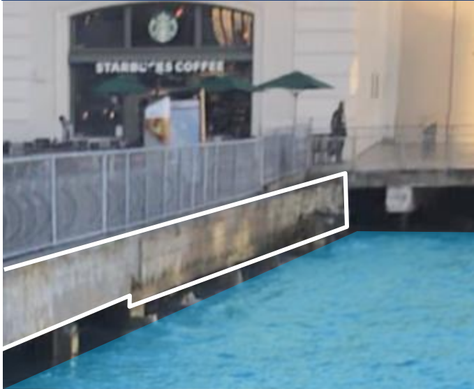
WHARF TODAY AT CURRENT WATER LEVEL
