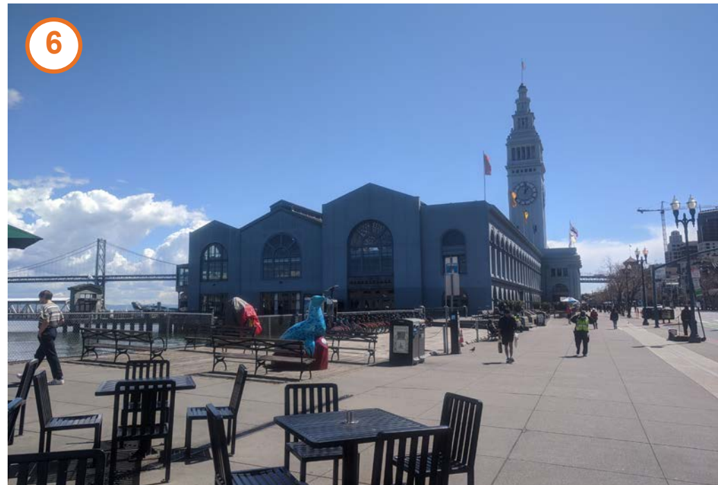
Pier 3 - South - Looking South
