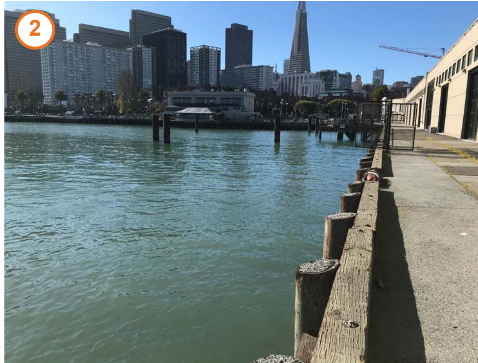
Pier 9 - Midway on Pier
