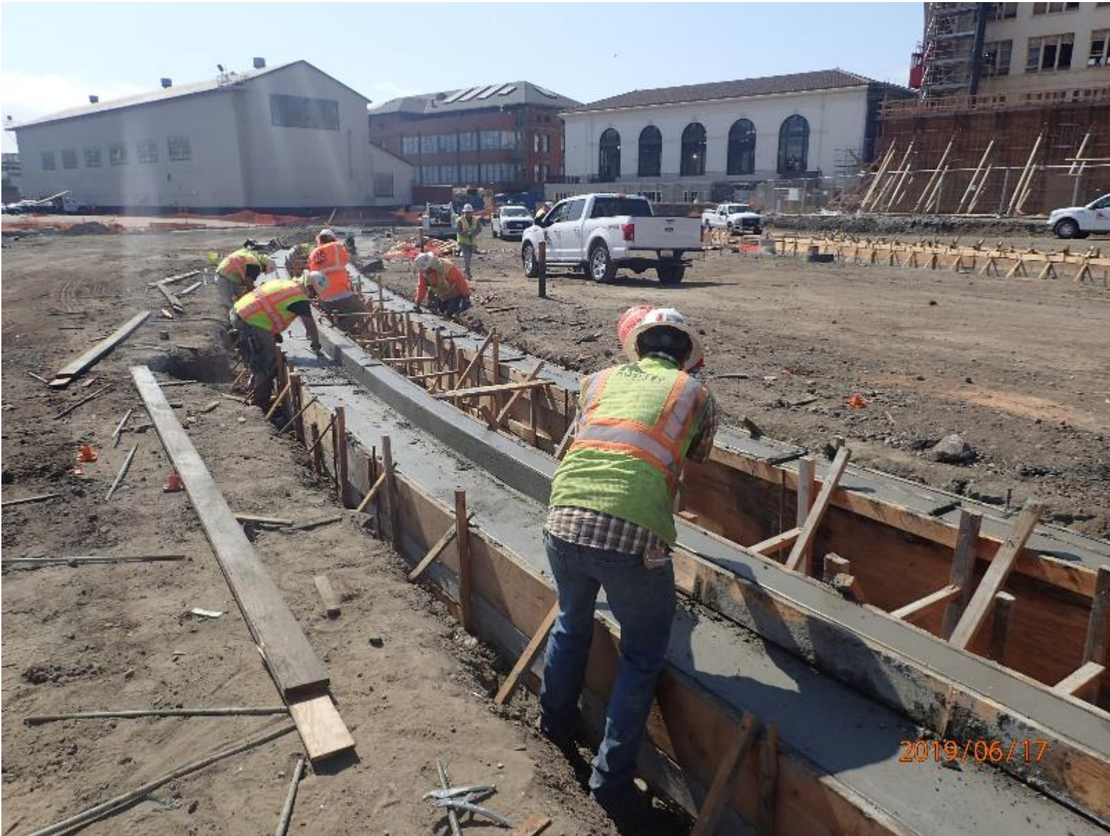
Figure 9: June 2019, Forming 19th St. Parking Lot Curbs
