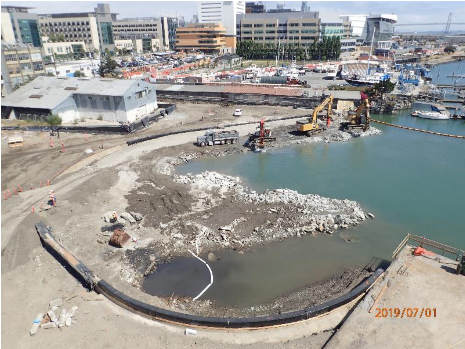
Figure 12: Beach Area Demolition – July 1, 2019 (Looking North)
