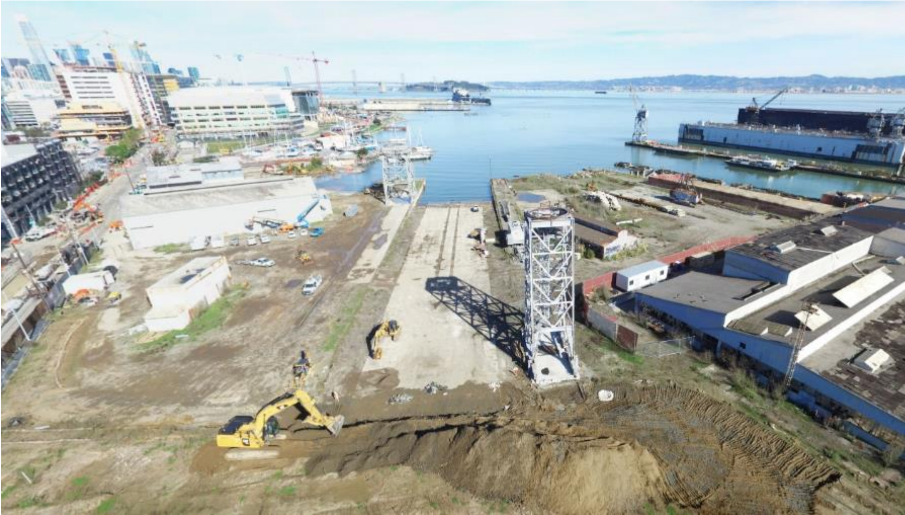
Figure 2: January 2019 (1 st month of construction) - Looking North east from Parking Lot
