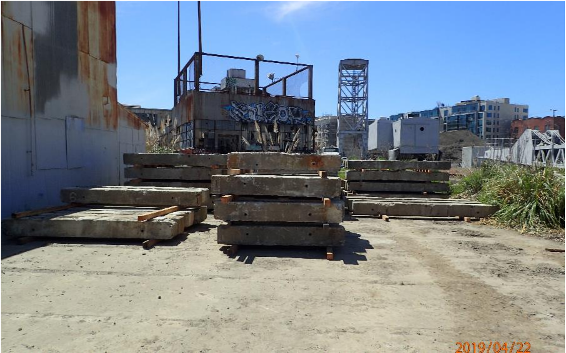
Figure 10: Cribbing Units sorted for custom site furnishings, April 2019
