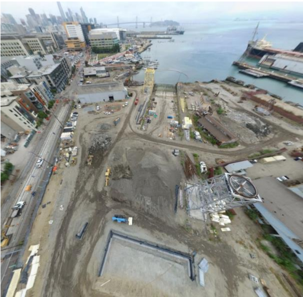
Figure 4: July 2019 (7 th month of construction) – Looking North from Parking Lot
