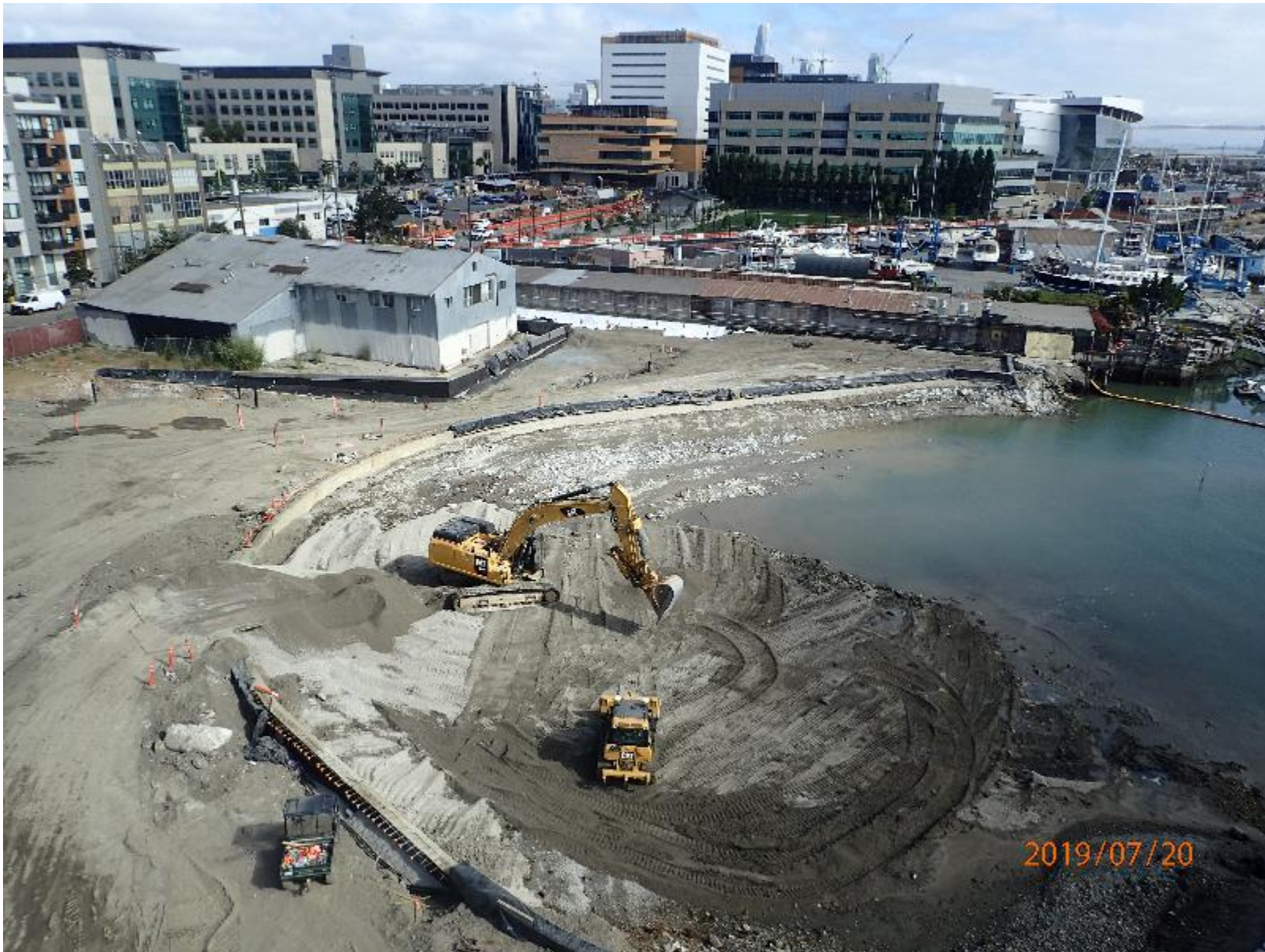
Figure 13: Beach Area Demolition & Sediment Cap Construction – July 20, 2019 (Looking North)
