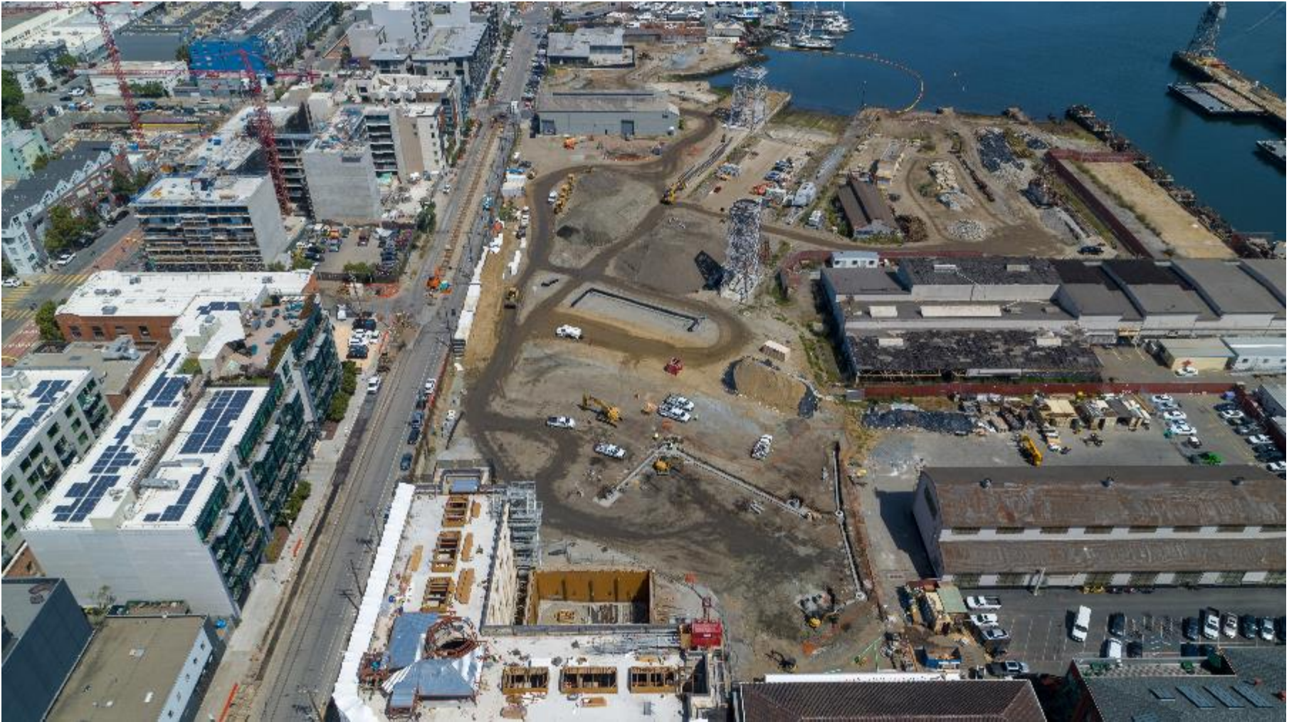
Figure 3: April 2019 (4th month of construction) - Looking North from Parking Lot
