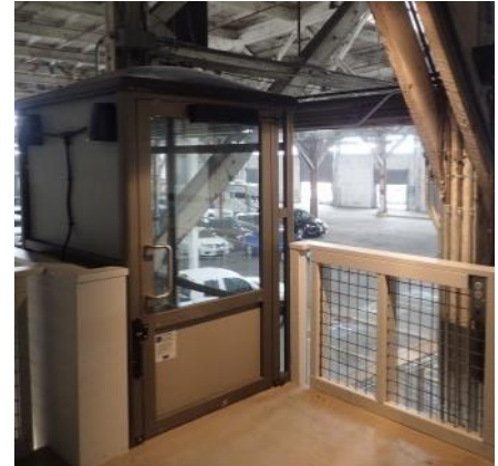
Figure 8: New ADA lift at Pier 31
