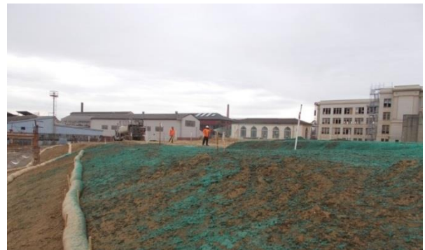
Figure 15: Site preparation work at future Crane Cove Park
