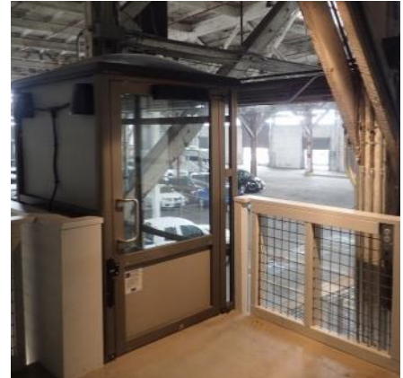
Figure 8: New ADA lift at Pier 31
