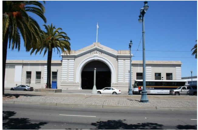
Figure 23: Pier 19 Bulkhead Building
