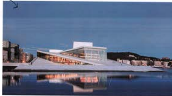
Oslo Opera House, Norway
