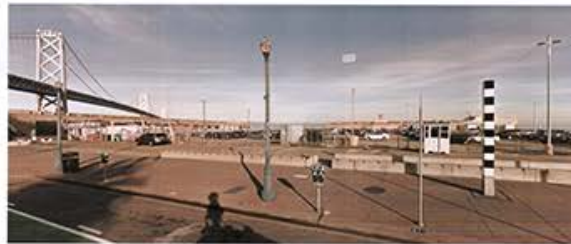
With this option, the fence, parking lot, and Red's Java House would be removed.
