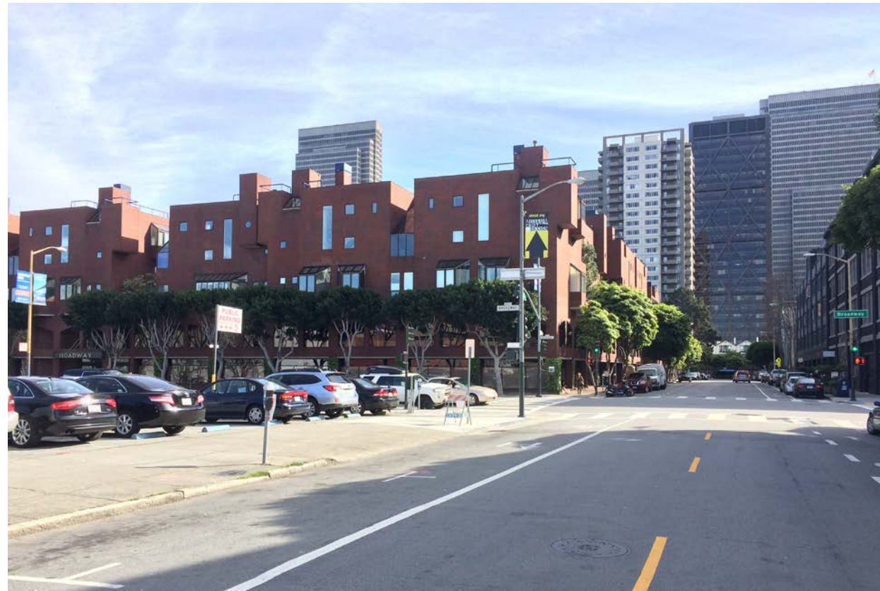
VIEW 1 LOOKING SOUTH ON FRONT STREET
