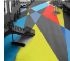
2 THERMOPLASTIC PAVEMENT COATING (ACCENT)
