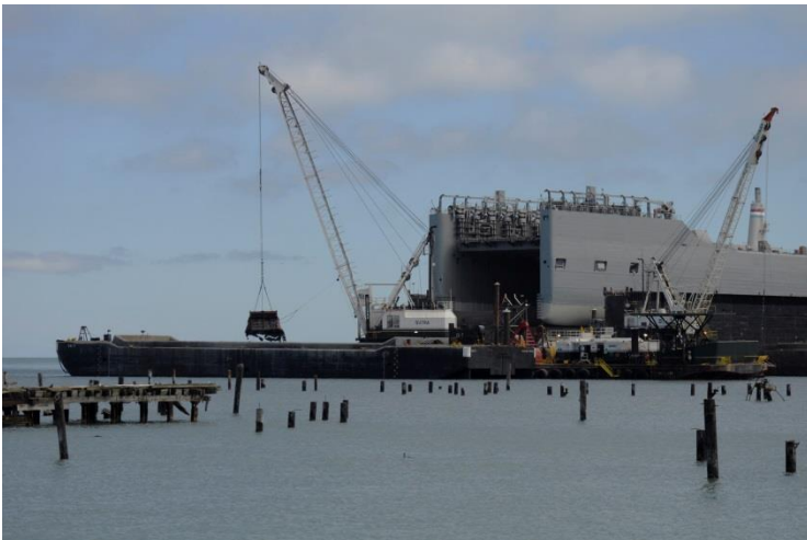
Figure 19: Prior dredging of Central Basin
