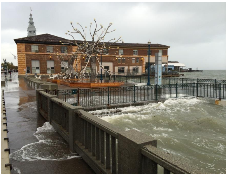
Figure 5: Flooding along Embarcadero during a king tide
