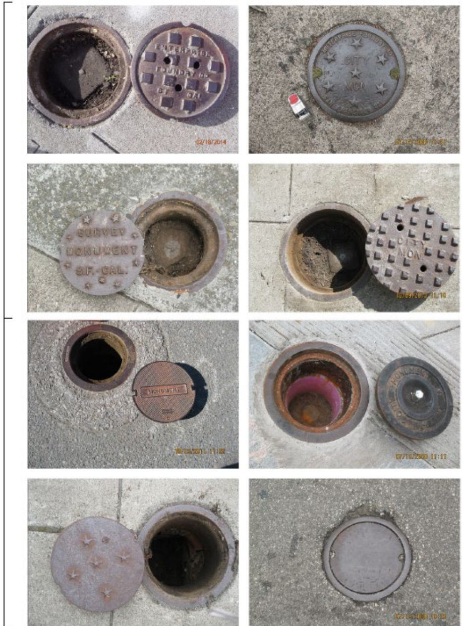
Typical Monuments with Well Casings
