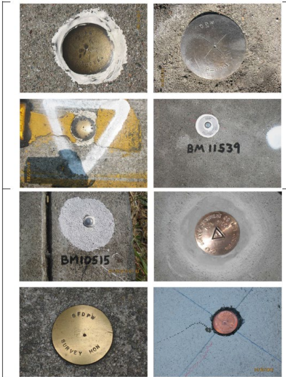
Figure 2 Typical Surface Monuments
