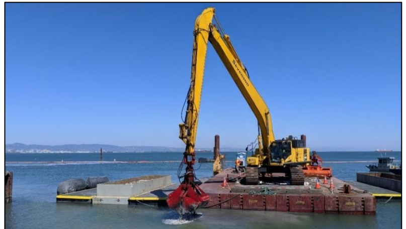
Example of offshore material dredging work
