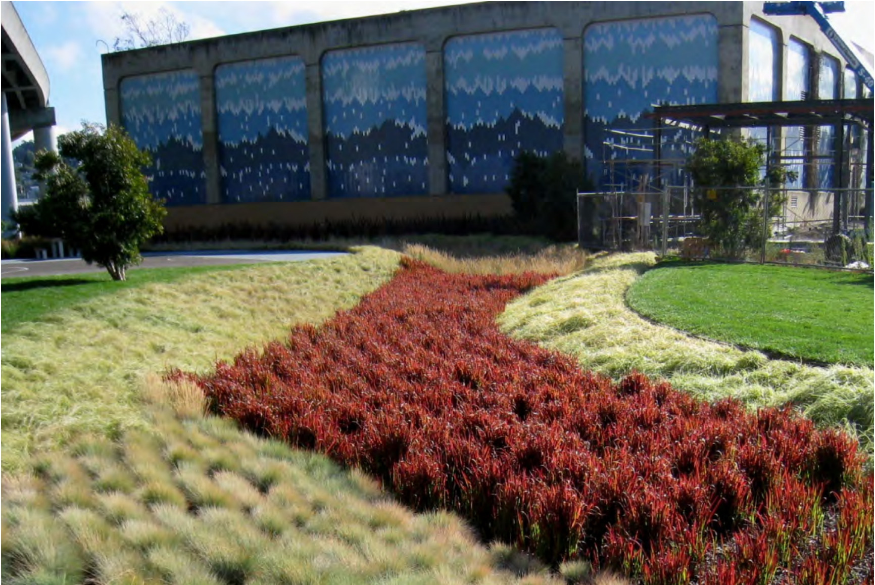
A swale in front of the San Francisco Public Utilities Commission's Channel Pump Station slows and treats stormwater before entering the Bay. Photo: SFPUC
