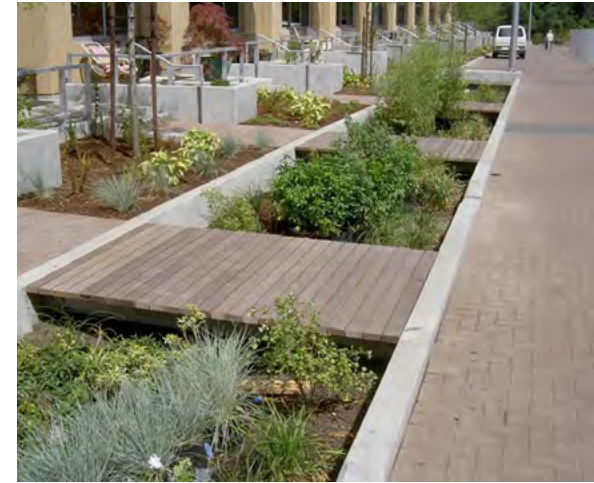
Rain gardens along Portland's waterfront provide functional greening elements. Photo: Ken Kortkamp
