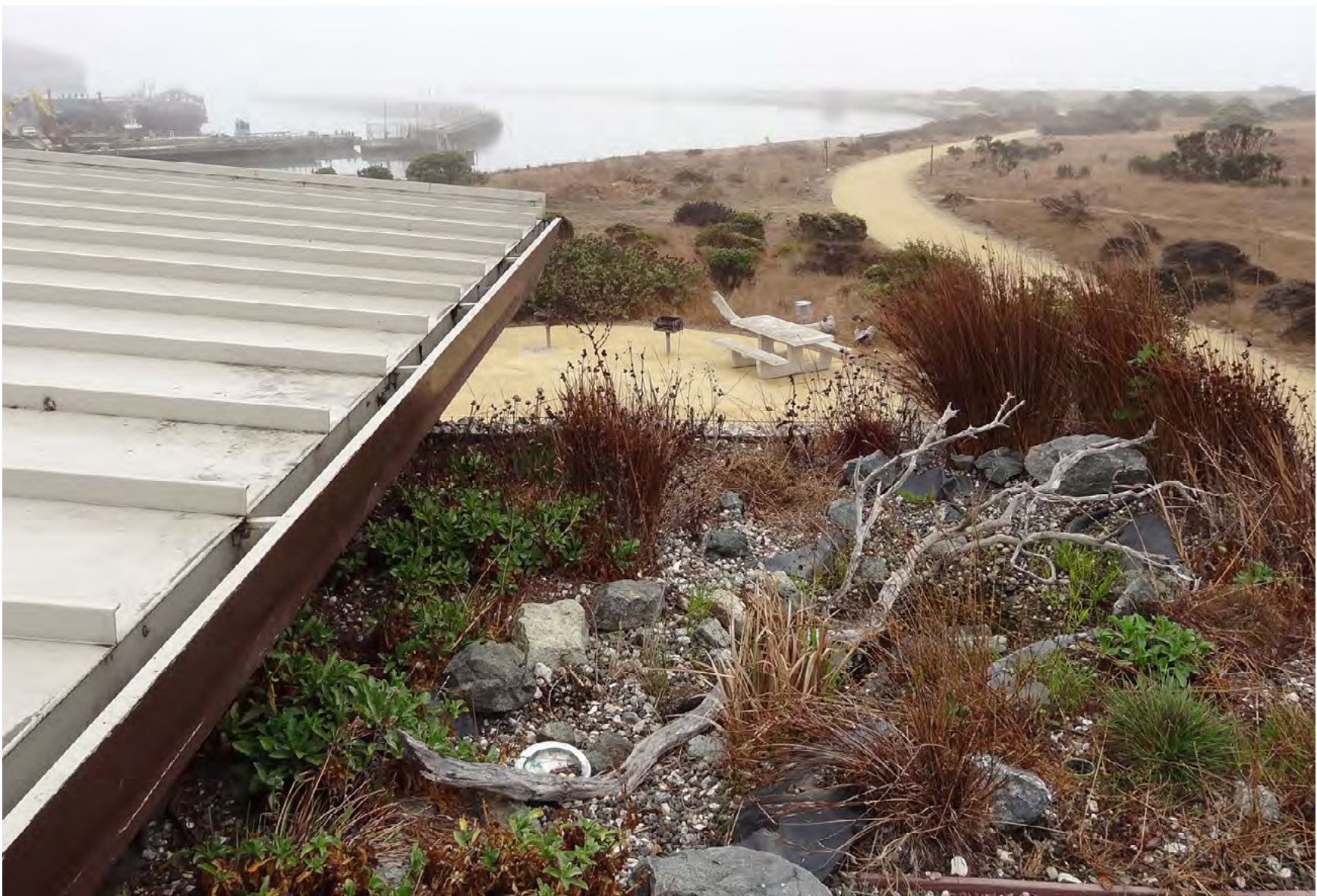
A vegetated roof and other LID features at the Eco-Center at Heron's Head Park help illustrate sustainable design practices to students in San Francisco's Bayview-Hunters Point neighborhood. Photo: Rosey Jencks
