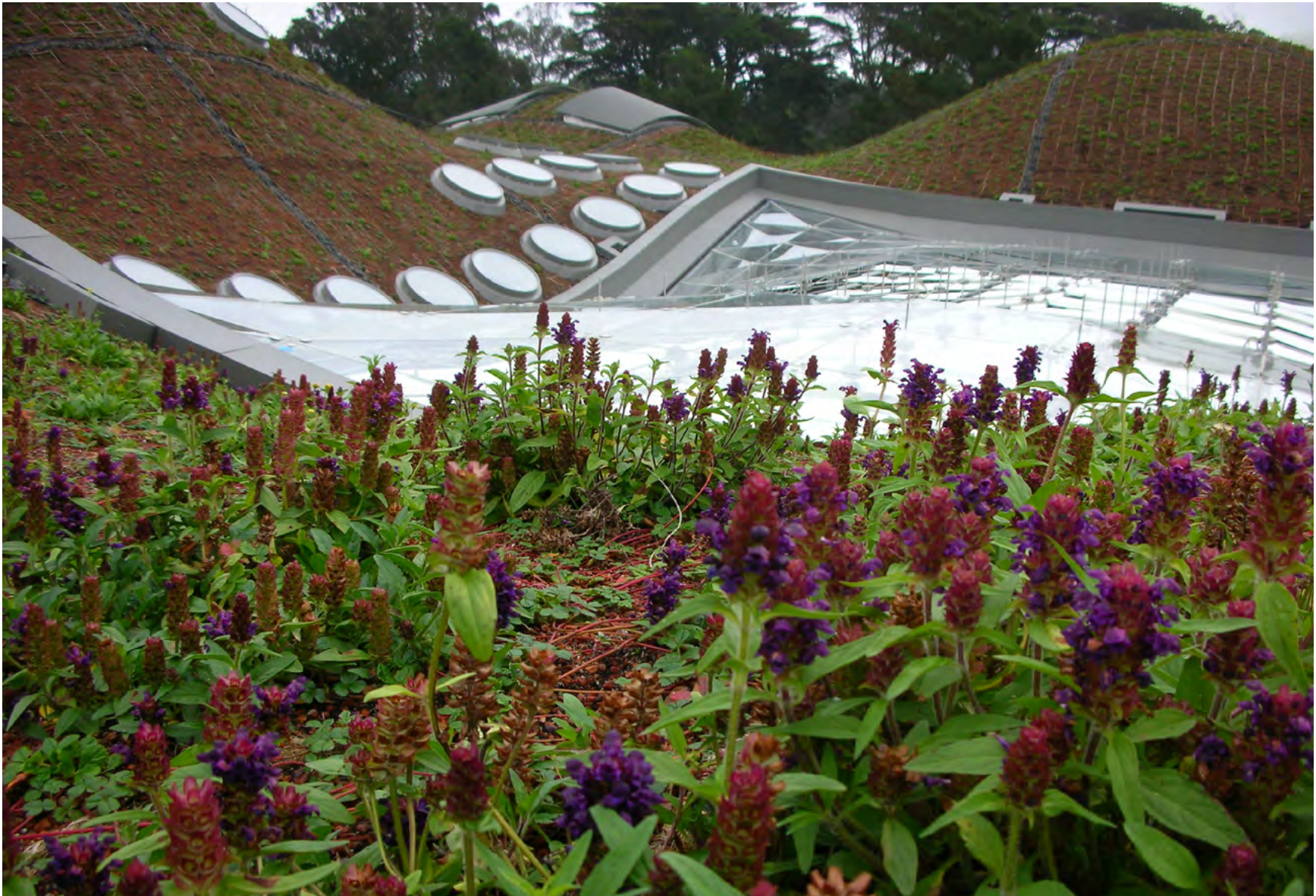
The Academy of Sciences in Golden Gate Park is a LEED Platinum building and includes a 2.5-acre vegetated roof. Photo: Rana Creek – Living Architecture
