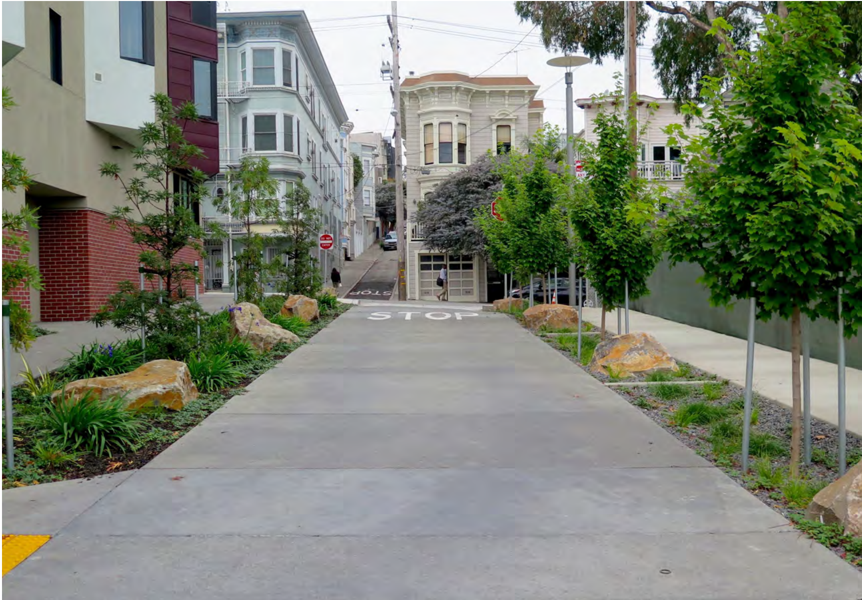
Hickory Street in San Francisco, CA is lined with bioretention on each side. Photo: Krystal Zamora
