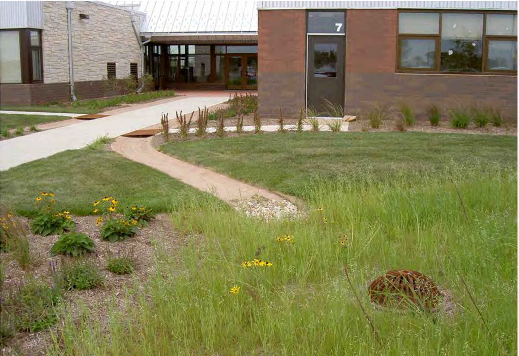
An impervious gutter directs roof runoff to a rain garden. Photo: Ken Kortkamp
