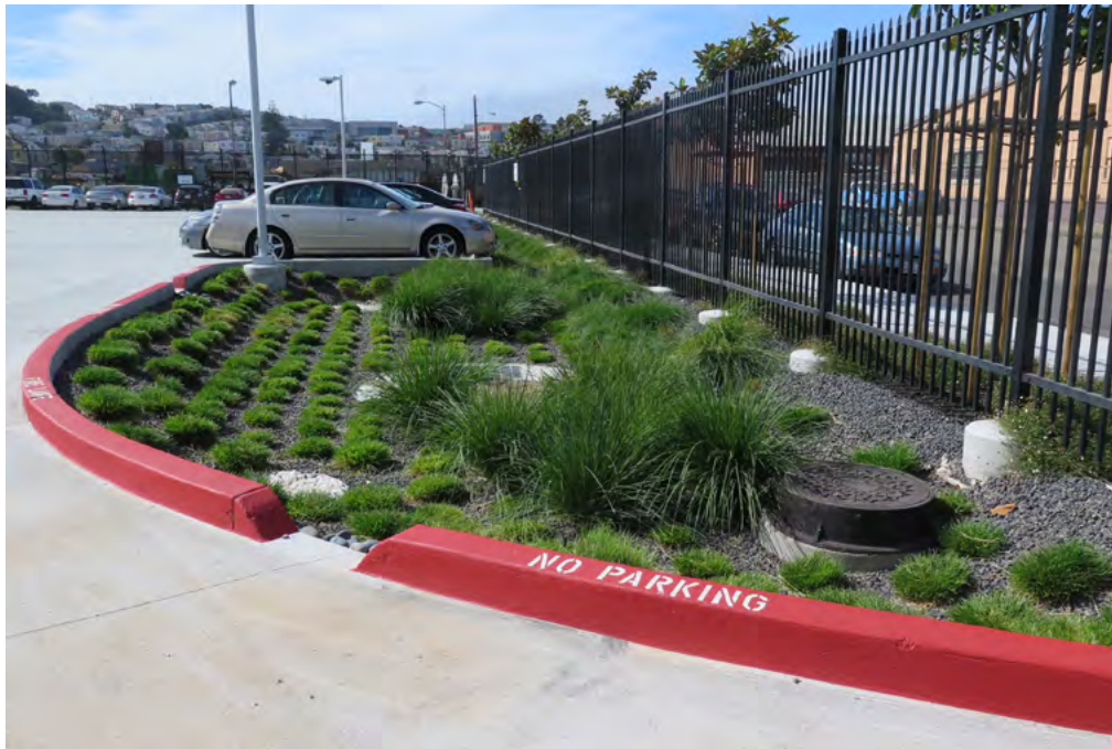
Bioretention reduces stormwater runoff in a parking lot at an industrial site in San Francisco. Photo: Krystal Zamora
