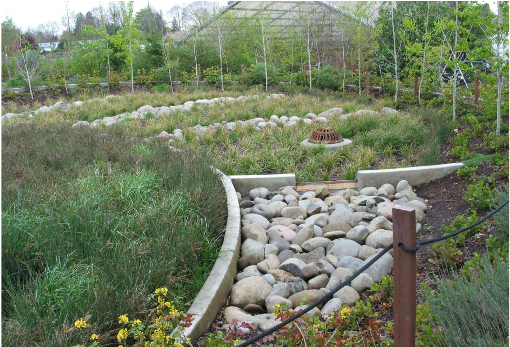
A rain garden at Glencoe Elementary in Portland, Oregon reduces stormwater flows to Portland's wastewater collection system. Photo: Rosey Jencks
