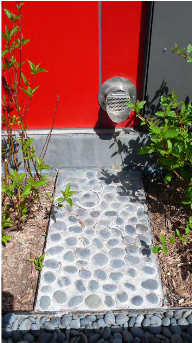
Fire Station No.1 in San Francisco met the SMR with bioretention and permeable concrete. Photo: Ken Kortkamp
