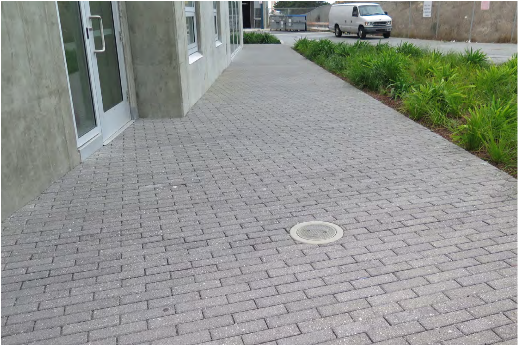
Permeable pavers contribute to this projects compliance with the SMR in San Francisco. Photo: Krystal Zamora
