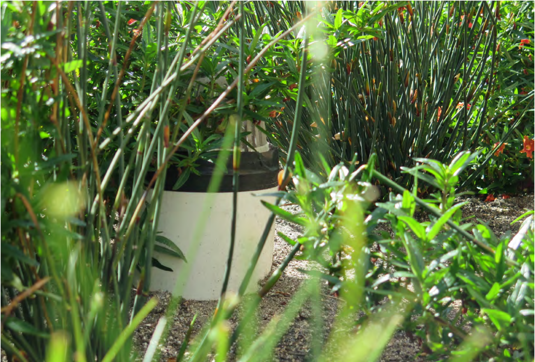
Modified Compliance was allowed for this multi-use building in the Mission District of San Francisco, which was constrained by Type D soils. Lined bioretention planters and rainwater harvesting were implemented to achieve the modified performance requirements Photo: Krystal Zamora
