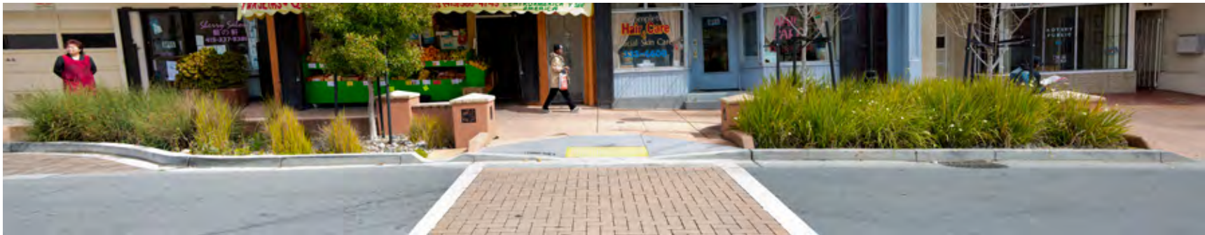
The Leland Ave Streetscape Improvement Project created one of the first streets to include green infrastructure in San Francisco, featuring bioretention and permeable pavement. Photo: Robin Scheswohl
