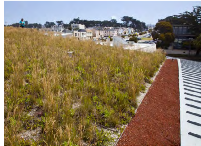
The vegetated roof at the Ortega Branch Library in San Francisco includes an Ortega Living Roof Cam that streams on their website. Photo: Robin Scheswhol
