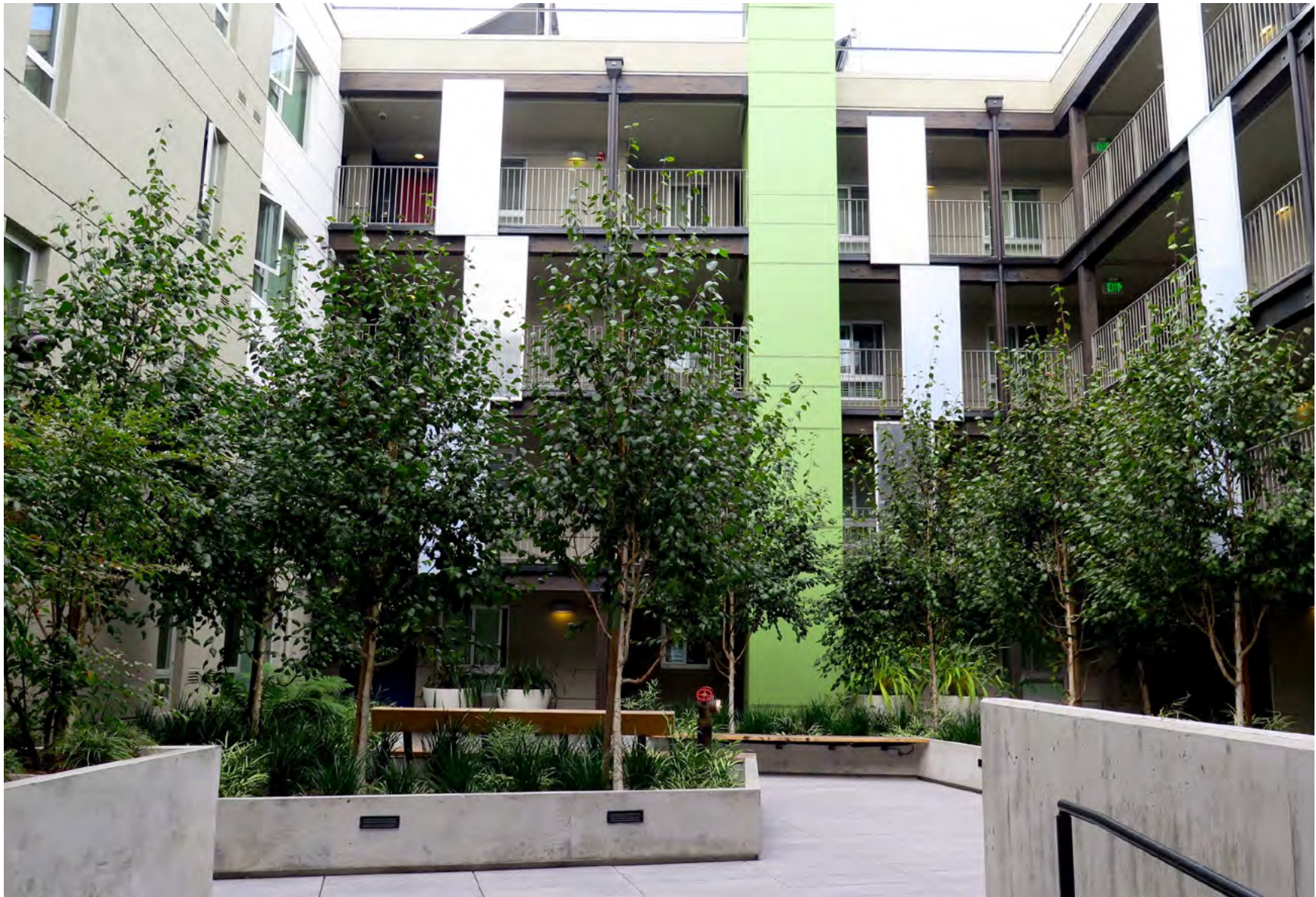
Bioretention planters are a central feature in a courtyard area. Photo: Krystal Zamora
