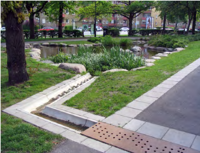
Conveyance features, such as this trench drain and runnel, can be used to move stormwater between treatment controls. Photo: Rosey Jencks
