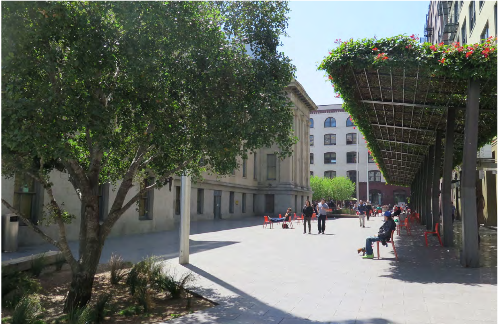
Mint Plaza in San Francisco is an example of how LID can be integrated into an ultra-urban setting. The design includes rain gardens, permeable paving, and a subsurface infiltration gallery. Photo: Krystal Zamora
