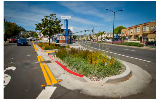
This joint project between the San Francisco Public Utilities Commission and Department of Public Works added bioretention planters as well as pedestrian, traffic, and bicycle improvements to Cesar Chavez St. Photo: Robin Scheswhol
