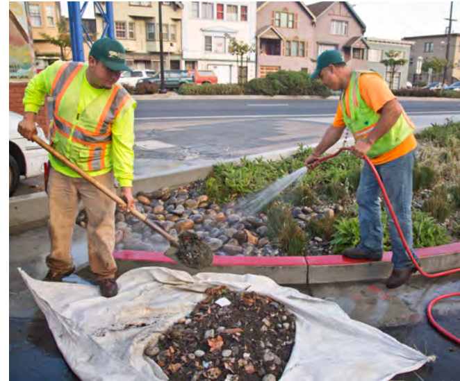
Maintenance workers remove sediment from a sediment basin in a bioretention planter on Cesar Chavez St in San Francisco. Photo: Robin Scheswohl
