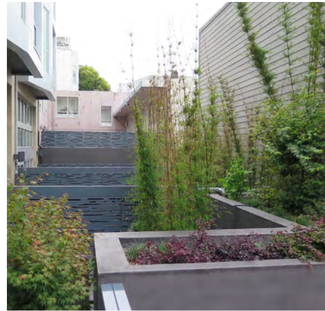
Bioretention planters are featured in private patios of a condominium development in San Francisco, CA.
