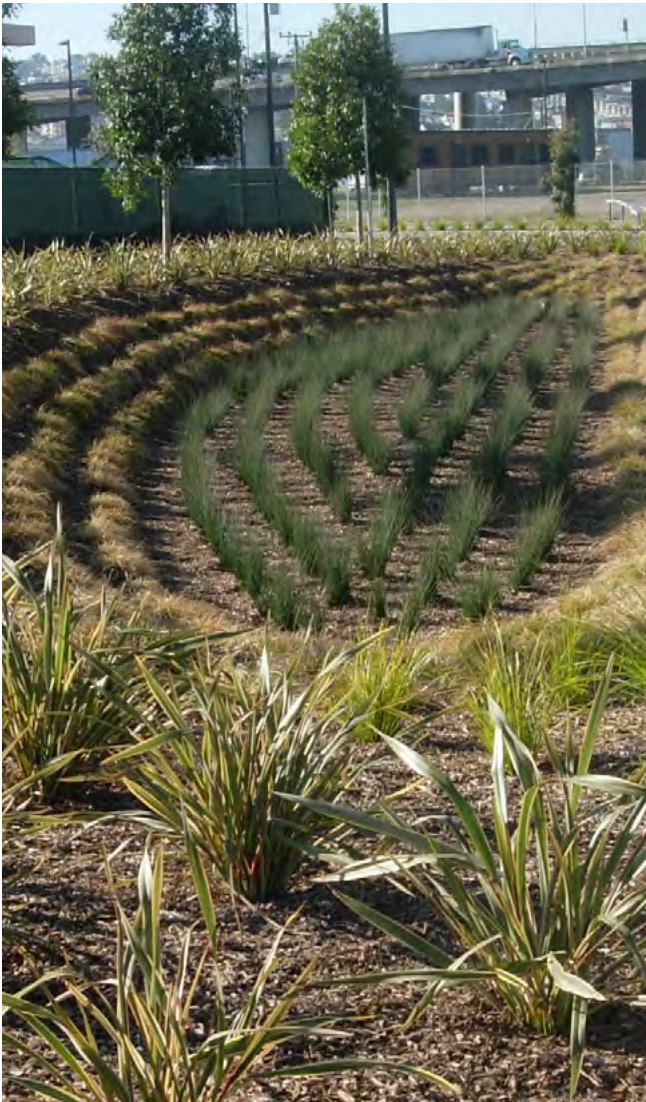
The Mission Bay traffic circle in San Francisco, CA manages stormwater from adjacent streets. Photo: Urban Watershed Management Program
