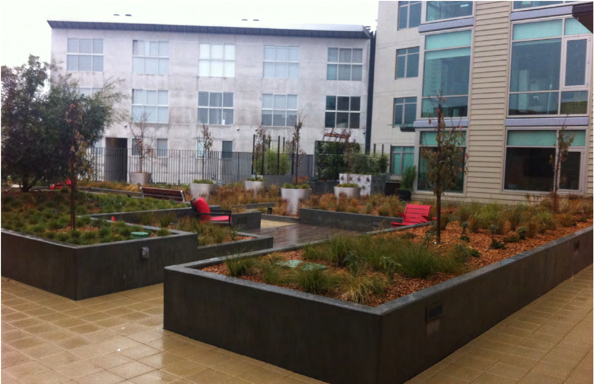
The Whole Foods building on Market St in San Francisco uses recycled water to water the planters on its rooftop patio. Photo: Ken Kortkamp
