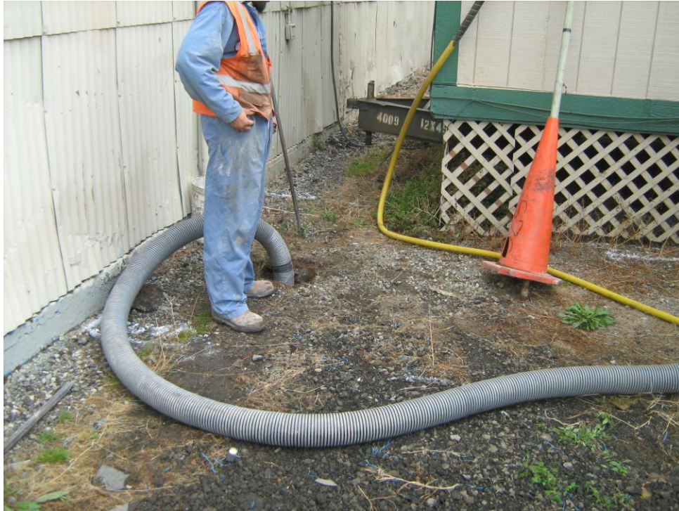
Photograph 12 – Boring area near suspect vent pipes south of Building 49
