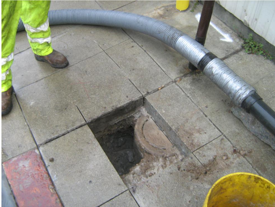
Photograph 6 – Concrete valve box beneath sidewalk
