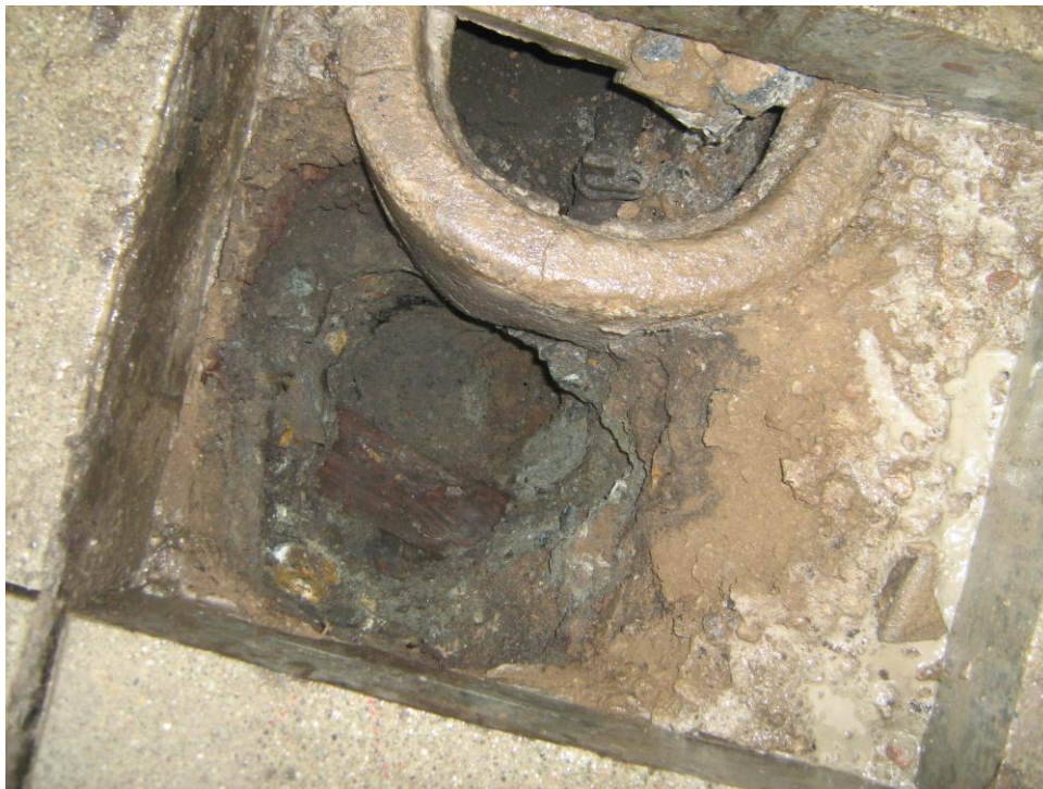
Photograph 7 - Air-knife boring located two feet west of suspect vent line. Photograph shows abandoned water valve inside valve box.
