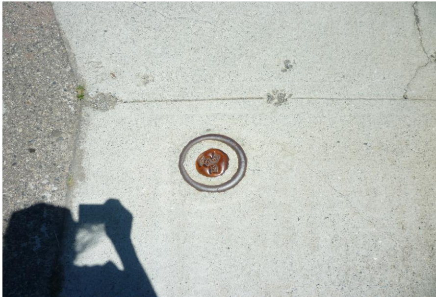
Photograph 4 - Unidentified circular metal object imbedded in concrete patch near the northeast corner of Building 11
