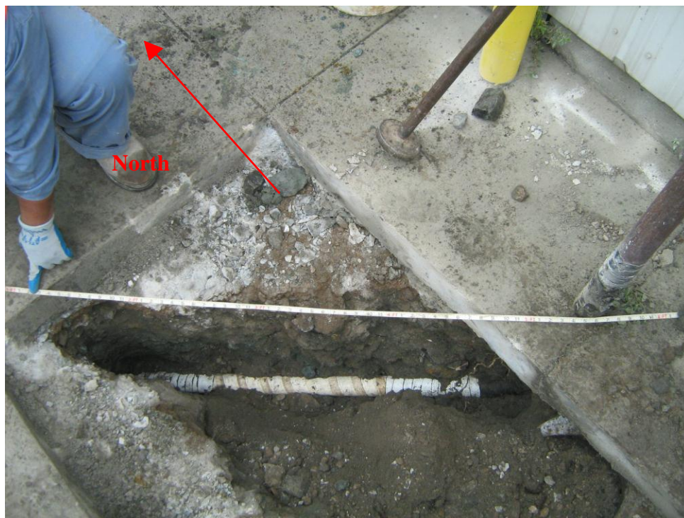
Photo 9 - Continuation of the suspect vent line plunging approximately 11 degrees in the northwest direction towards Illinois Street
