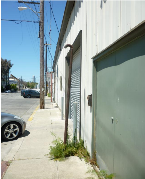
Photograph 1 - Suspected vent pipe located in sidewalk on east side of Illinois Street, in front of Building 49
