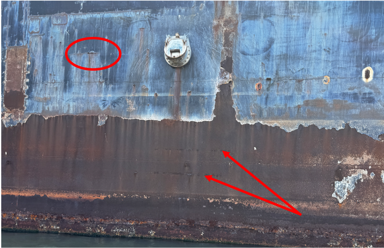
Photograph 31 - External view of side shell tears at Tank 29
