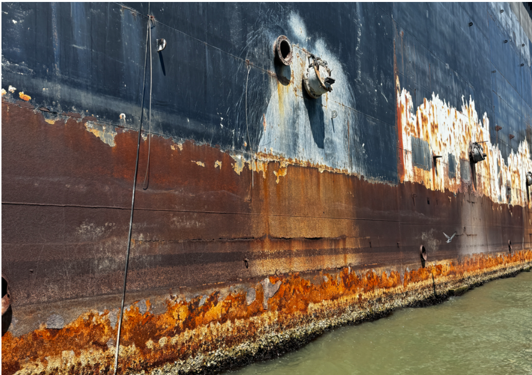
FIGURE 1 - TYPICAL CONDITION OF OUTBOARD SHELL (EAST/PORT)
