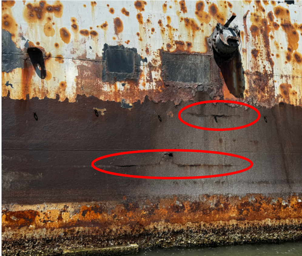
Photograph 15 - External View of Tank 16 side shell tear
