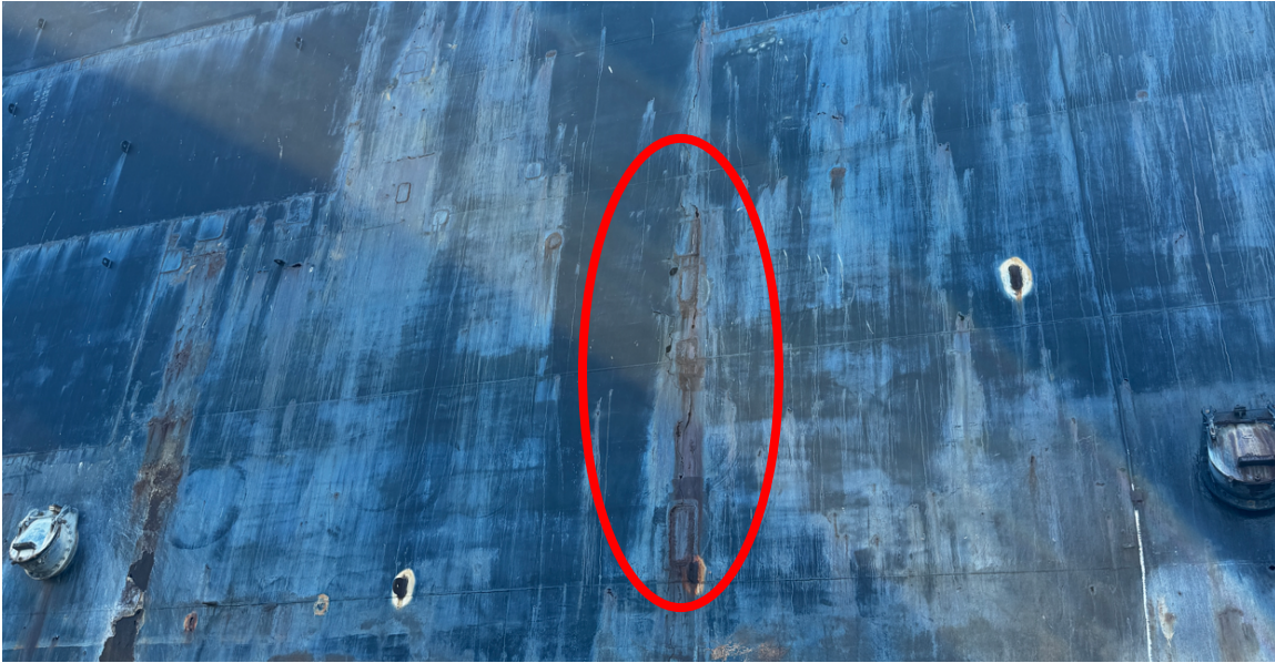
Photograph 33 - External view of vertical wing shell tear at Tank 29
