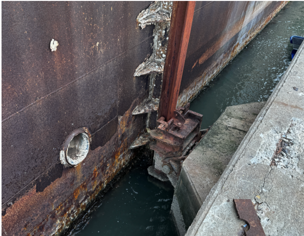
FIGURE 2 - TYPICAL CONDITION OF A MOORING POINT
