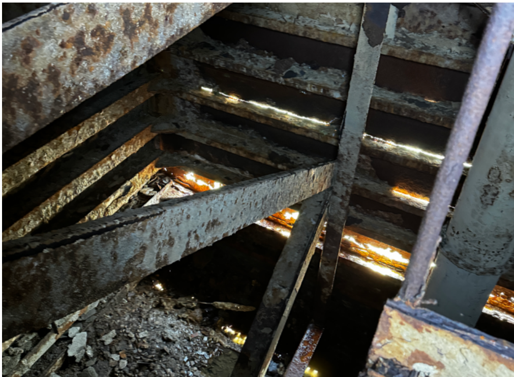
Photograph 2 - View of Tank 40 shell tears internally (FR 77-80)
