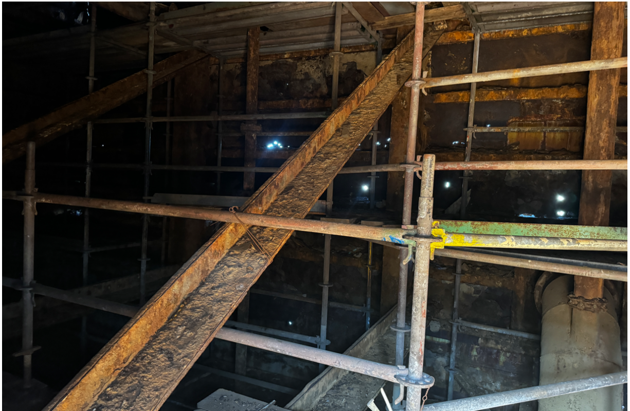
Photograph 29 - Internal view of pontoon deck level holes at Tank 23
