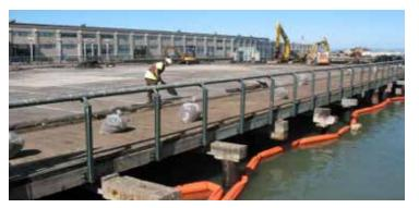
Floating boom is deployed around construction work to capture debris.
