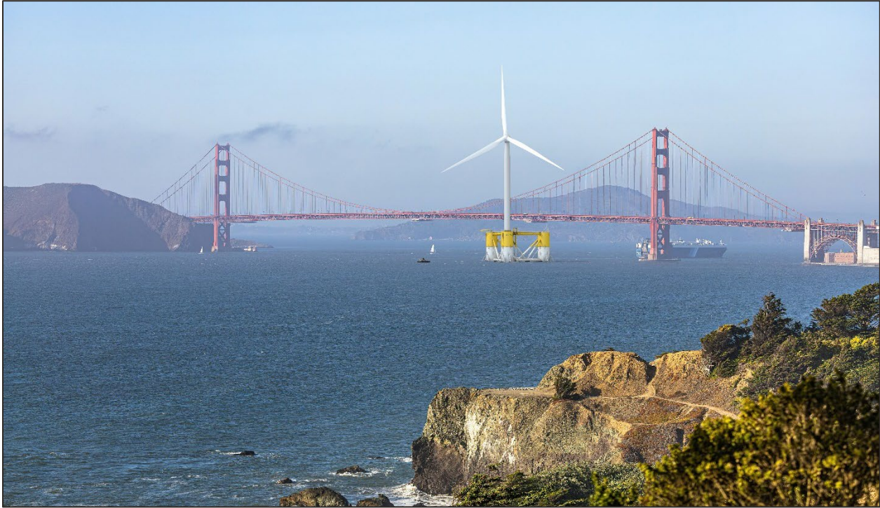
Figure 3: Rendering of offshore wind turbine near Golden Gate Bridge to highlight air draft restrictions.
