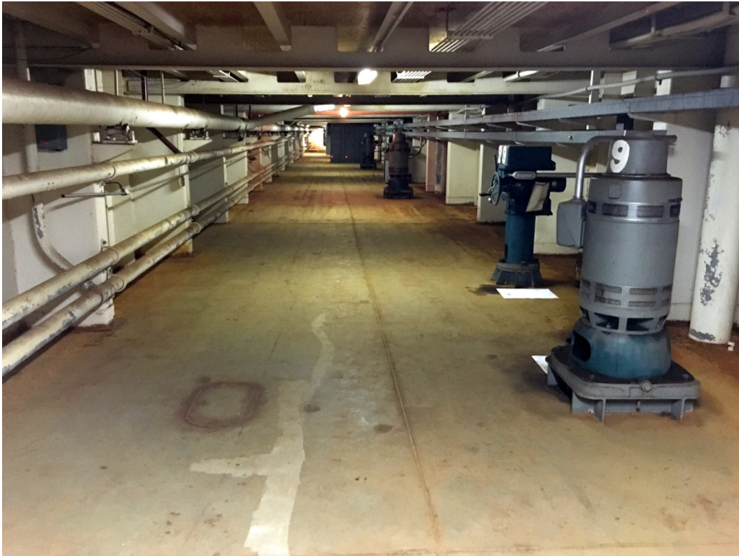
Photo 18: Typical condition of safety deck compartment.
