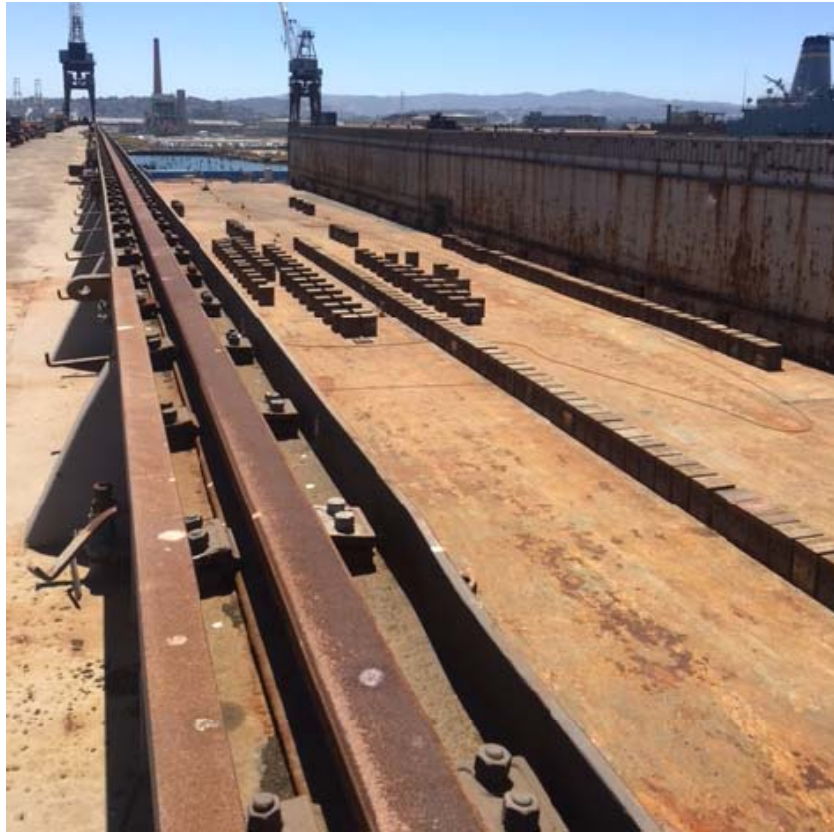
Photo 1: Drydock keel block set up.
