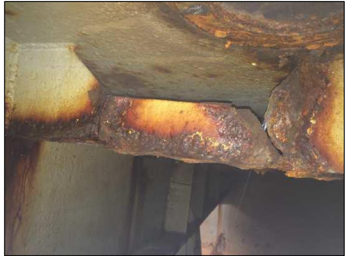
TYPICAL FRACTURE IN WAY OF CHANNEL CUT OUT SHOWN.
