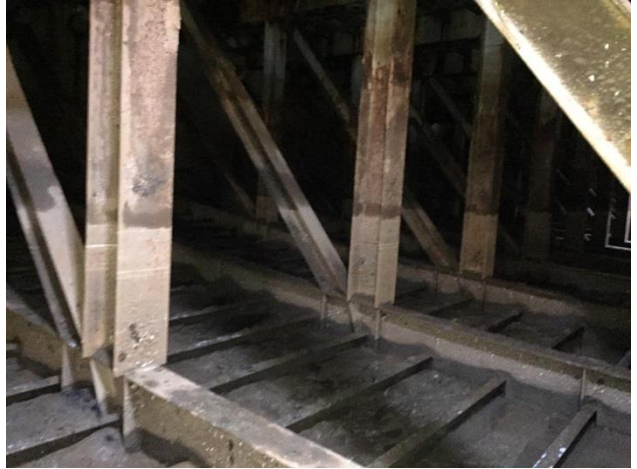
12. Braced frames at Tank 9
