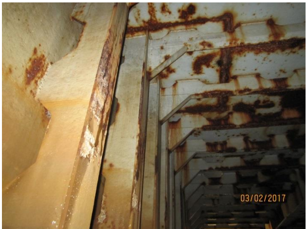
21. Wall stiffeners at Tank 6
