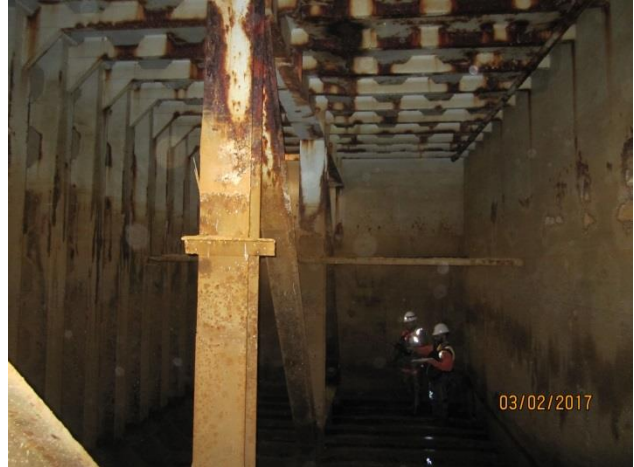
20. Roof stiffeners and braced frame at Tank 6
