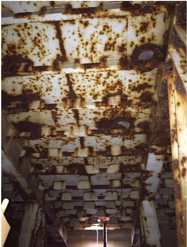
17. Roof stiffeners at Tank 5
