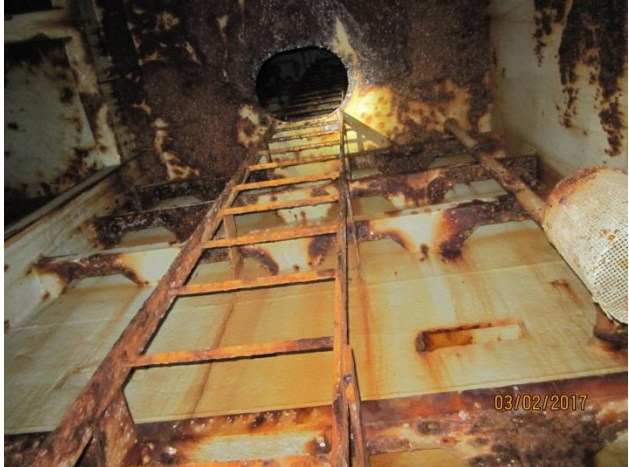
19. Ladder up wing wall at Tank 6
