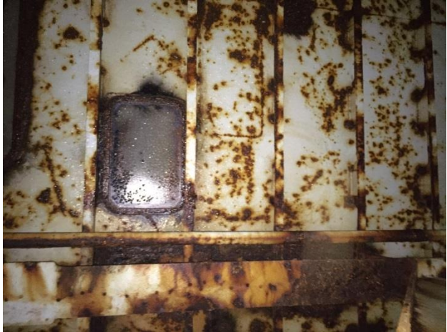
15. Roof stiffeners at Tank 6
