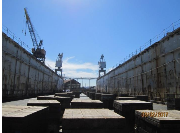
8. South view of support blocks and interior faces of wing walls
