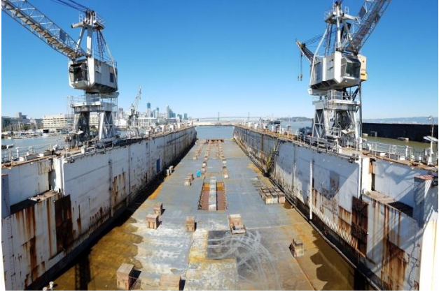
1. North View of along the length of Dry Dock EUREKA
