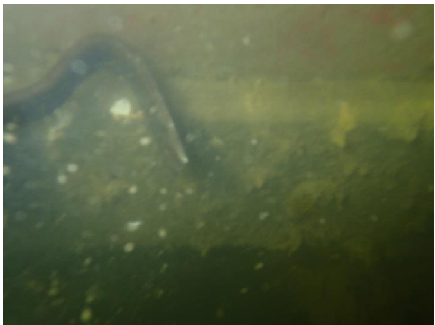
23. Removal of marine growth for inspection
