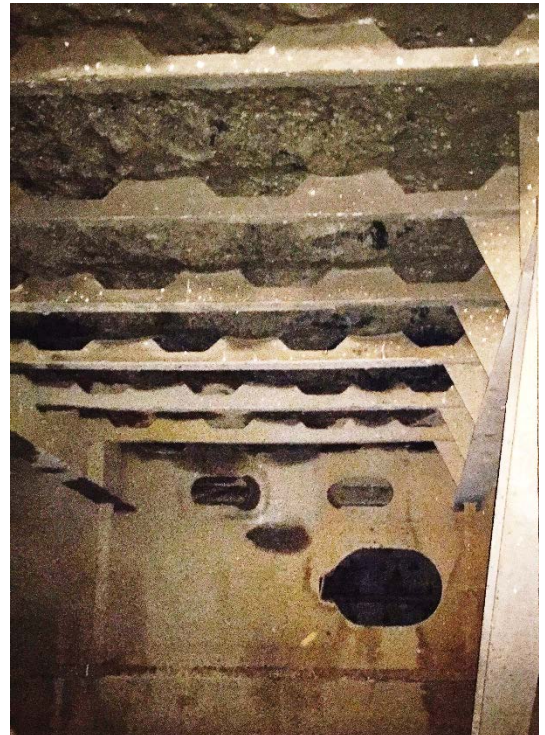
Figure 6: Undamaged Serrated Stiffener Example
