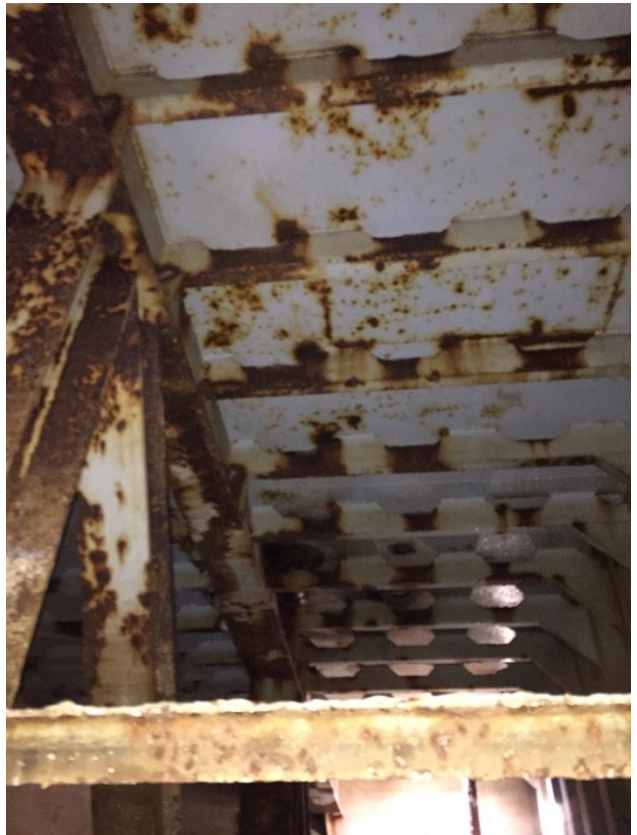
14. Roof stiffeners at Tank 6A
