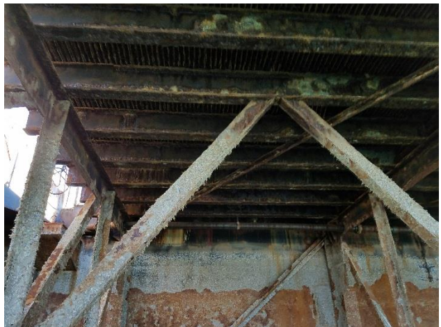
18. South apron, below
