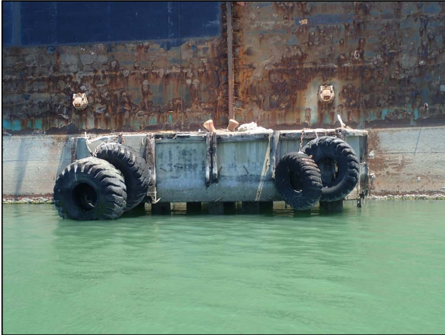
Photograph 5 : Overall View of Mooring Dolphin 2, Looking East.
