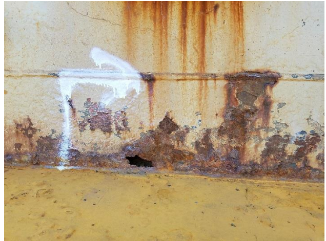
8. Inner shell at pontoon level with through hole
