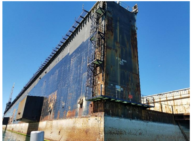
10. South end of west wingwall
