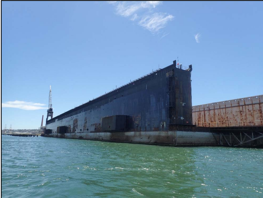
Photograph 3 : Overall View of the East Wingwall of Dry Dock 2, Looking Southwest.
