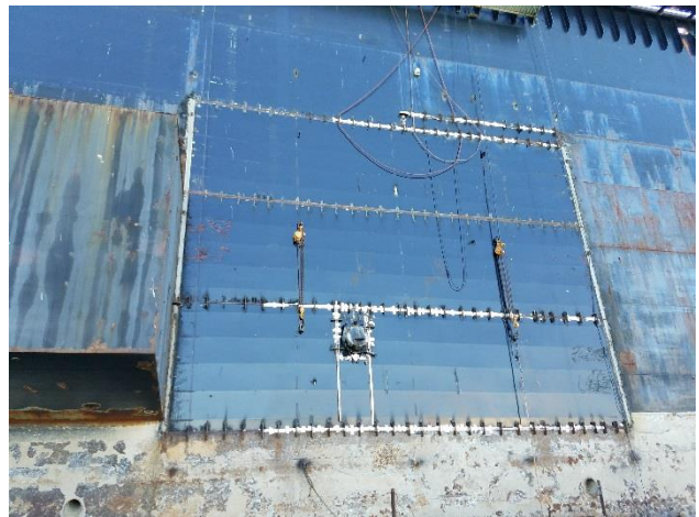
12. Recently replaced outer shell panels
