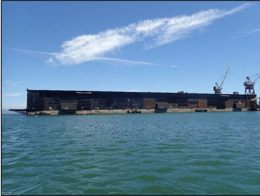
Photograph 1 : Overall View of Dry Dock 2, Looking East.
