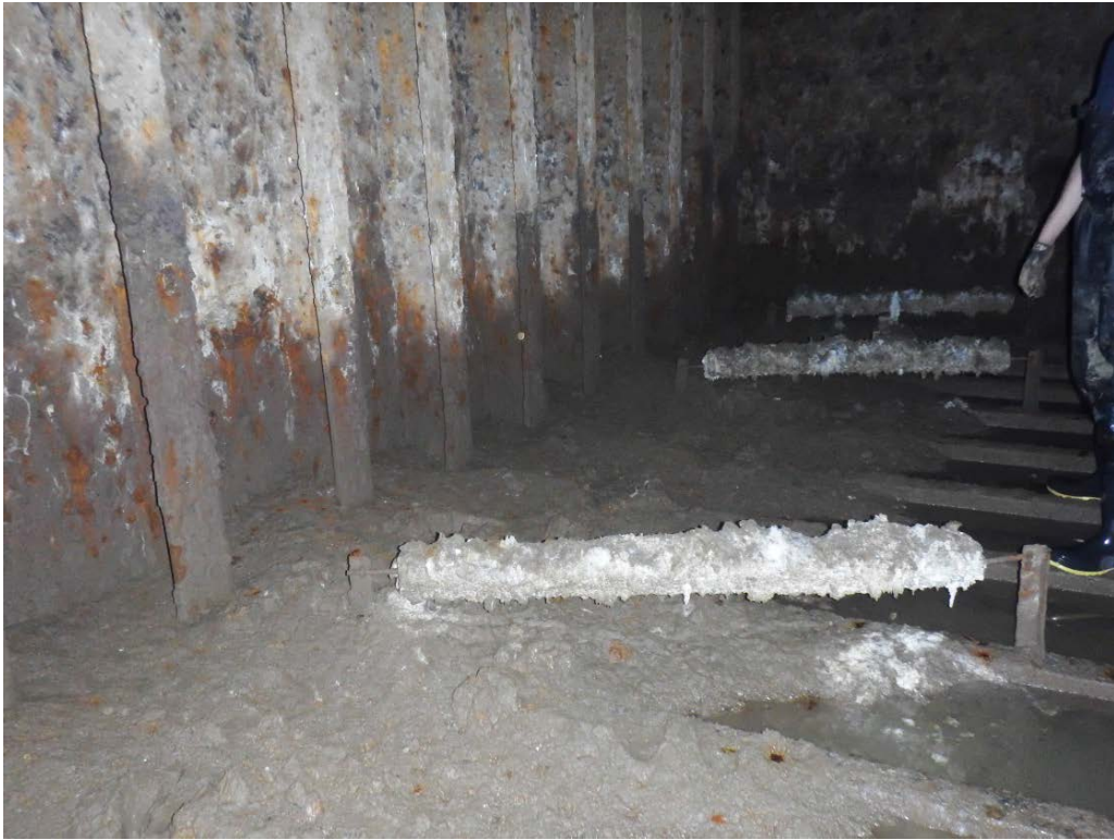
Figure 8: Typical condition of pontoon ballast tanks (Heger Dry Dock Inc.)
