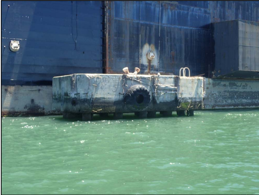
Photograph 7 : Overall View of Mooring Dolphin 4, Looking Southeast.
