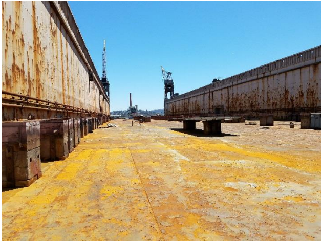
1. On pontoon deck, looking north
