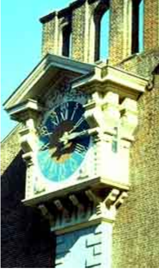
In the reconstruction of the clock tower at Independence Hall, the substitute materials used were cast stone and wood with fiberglass and polyester bronze ornamentation. Photo: NPS files.
