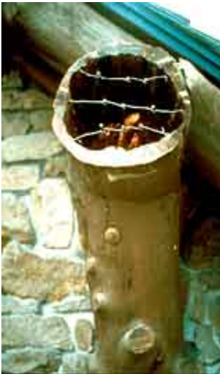
The core of a deteriorated wood outrigger was first drilled out. Photos (left and right): Courtesy, Harrison Goodall.
