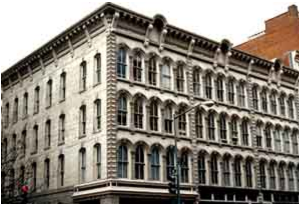
The historic cornice was successfully replaced with a fiberglass cornice. Photo: NPS files.
