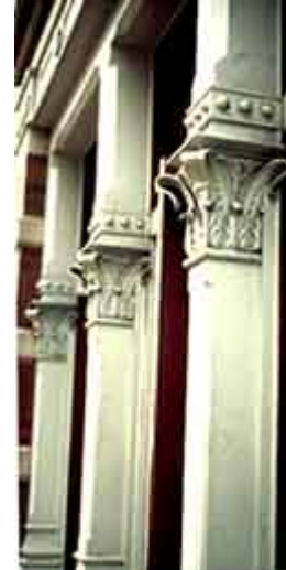
Cast aluminum has been used as a replacement material for cast iron. Photo: NPS files.
