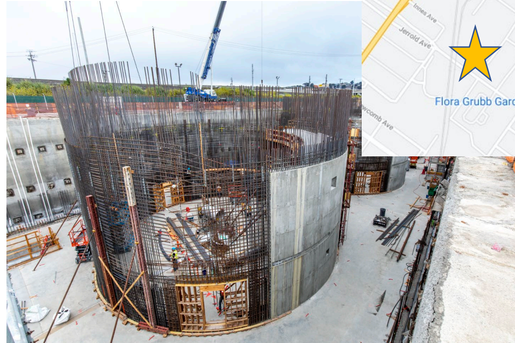
Rebar and concrete taking shape into one of the five new digesters.
