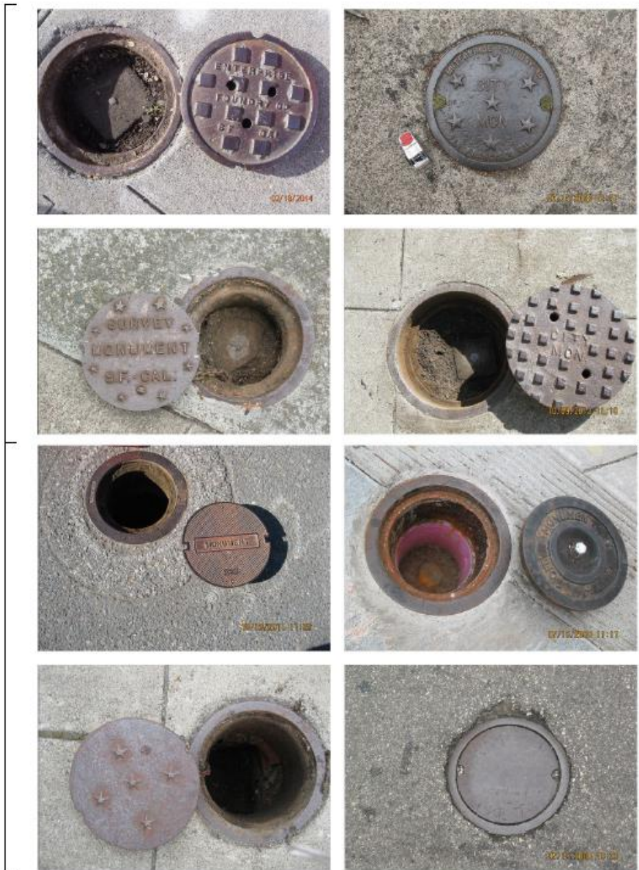
Typical Monuments with Well Casings
