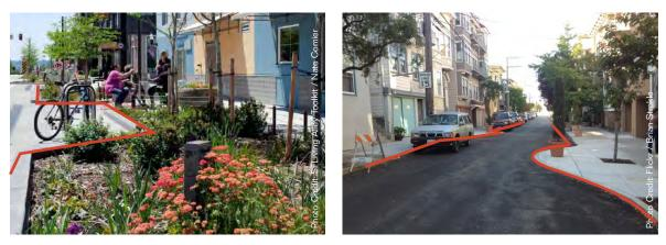
FIGURE 4.6.2: Example of Bulb-outs, Chicanes, and On-Street Parking
