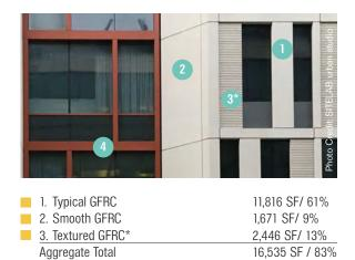
Note: Includes area recessed or projected up to the limit of measure (10' depth)
