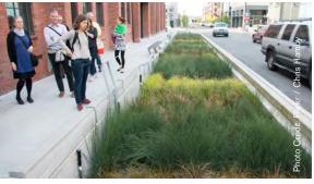
Sidewalk with Stormwater Planter
