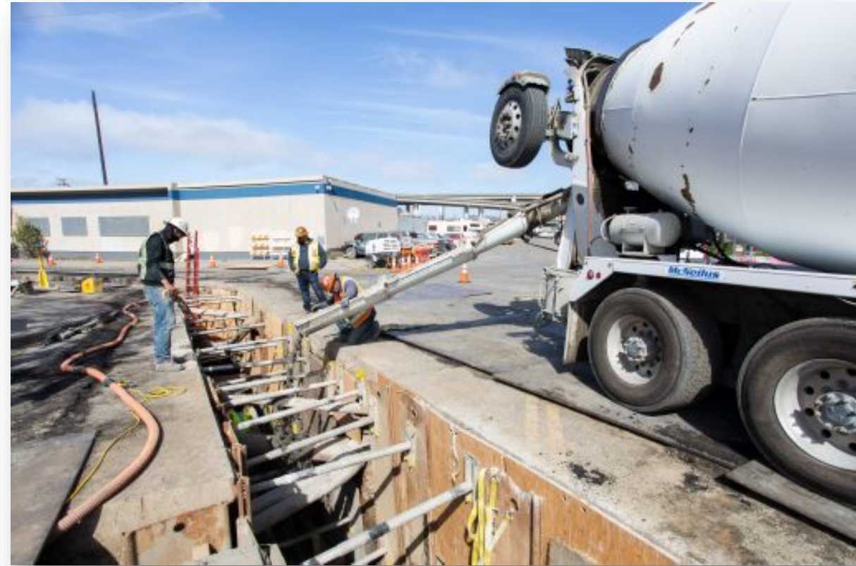
Pouring concrete for electrical conduits as part of the BCTD Project.
