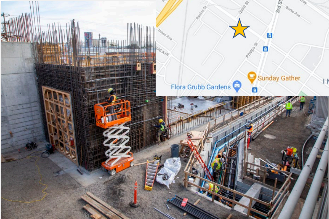
Construction of grit handling and duct bank.
