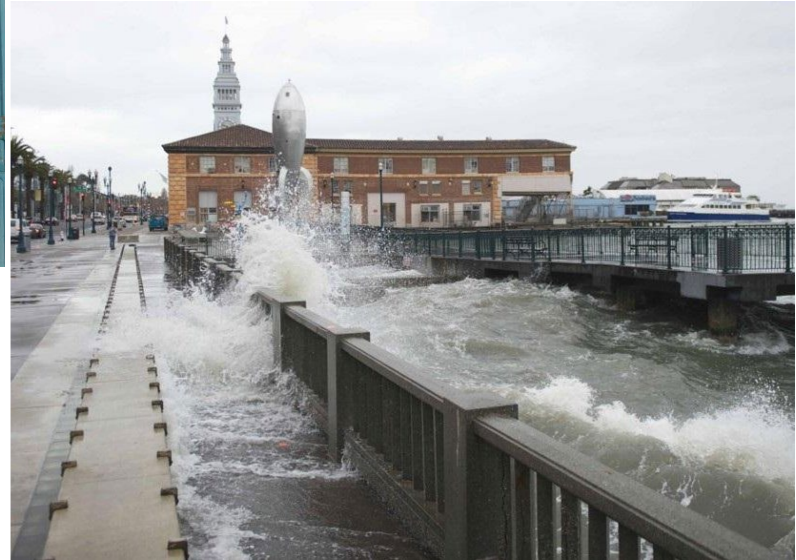
PIERS 30-32 & SEAWALL 330 CURRENT SEA LEVELS
