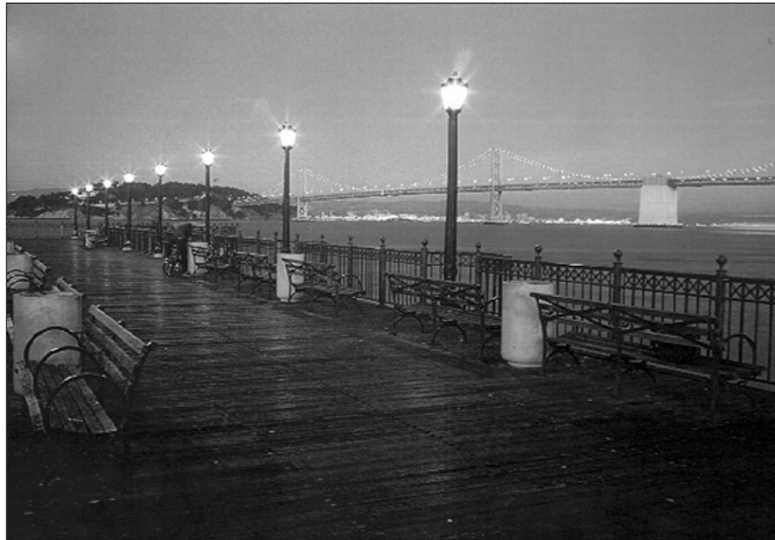
Pier 7 public access pier
