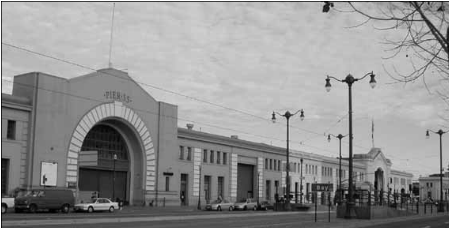
Pier 33 & 35 bulkhead & connector buildings near the foot of Bay Street
