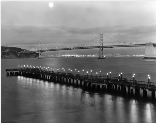
Pier 7 public access pier
