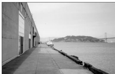
Piers extend out from the seawall edge. Shown above is Pier 9’s south apron.
