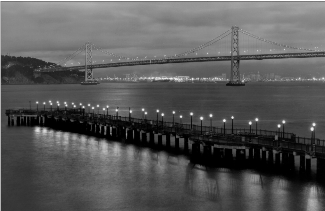
Pier 7 public access and fishing pier
