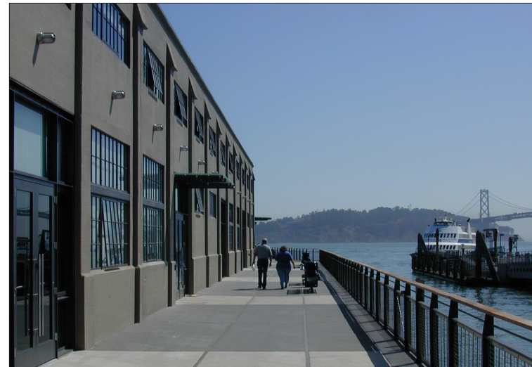
Pier 1 south apron
