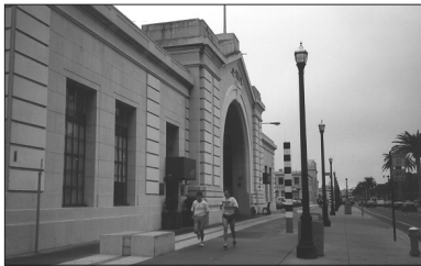
Pier 9 Bulkhead Building
