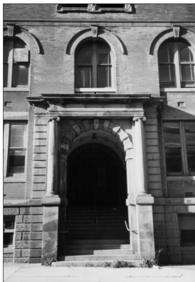
Entry to Building No. 102
