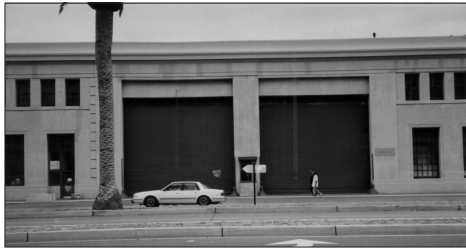
Potential opening in Bulkhead Connector Building 29 through service doors.
