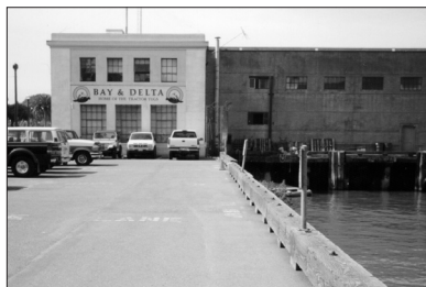
Wharves are structures that generally run parallel and adjacent to the seawall. Shown above is the wharf between Piers 17 and 19.
