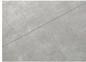
*CIP Concrete Natural Gray with Silica Carbide & Water Jet Finish
