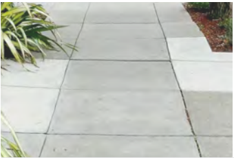
2 Concrete Sidewalk: SFPW Standard CIP Concrete
