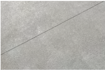
2a Upgraded Concrete Sidewalk Finish - Silica Carbide / Sandblast
