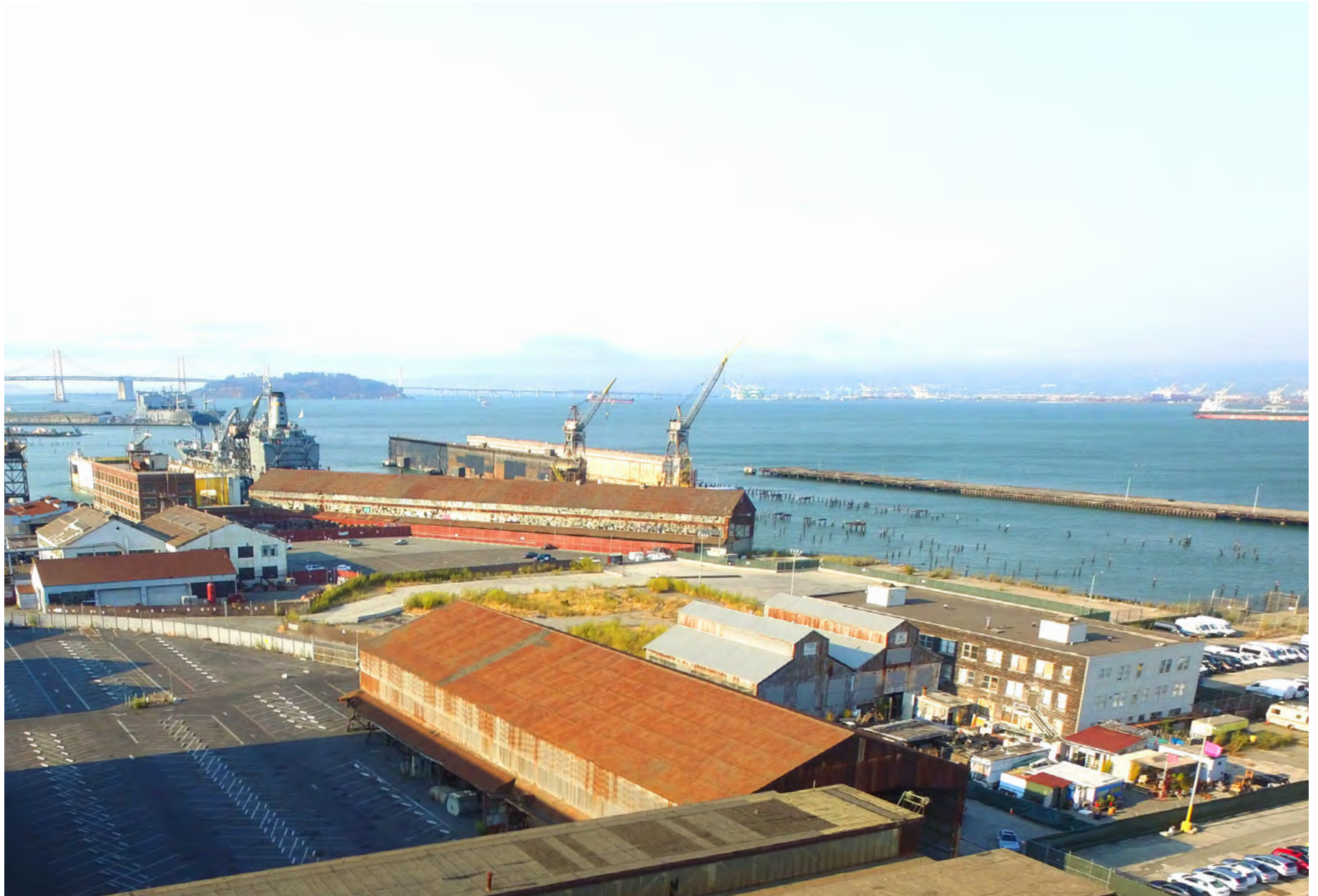
Overlooking existing Building 12 toward future location of Waterfront Street
