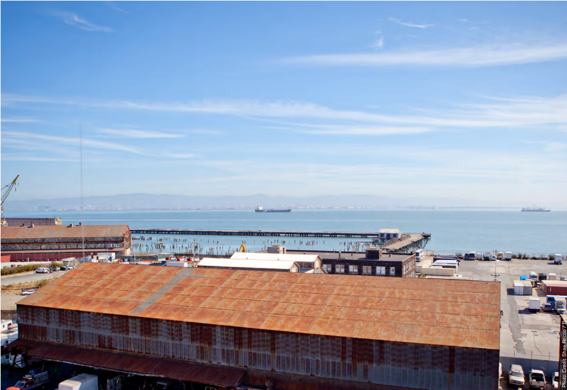
View from existing Building 2 toward future location of Waterfront St.
