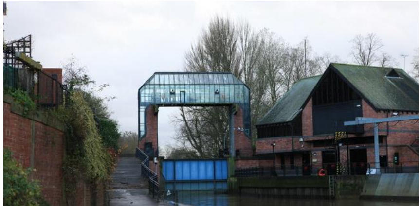
The Foss Barrier, a 16 tonne gate built in 1989, is lowered into the River Foss to stop the Foss levels from rising flood waters on the River Ouse - York, England ©Michael Jagger/Foss Flood Barrier/CC BY-SA 2.0
