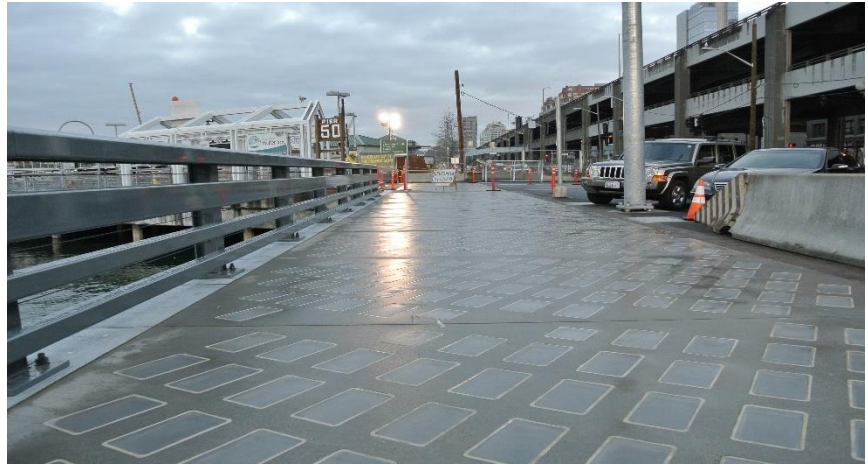
Seawall: Light Penetrating Sidewalk Installed - Seattle, WA. ©Seattle DOT via Flickr.com
