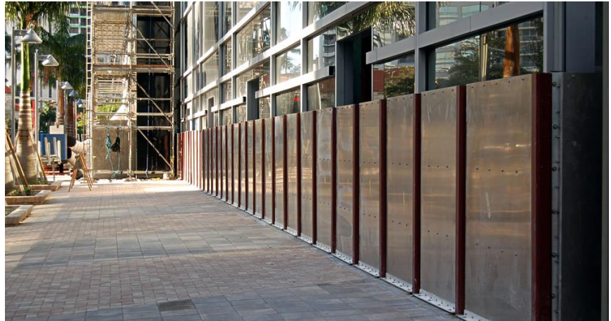
Post and panel installation in Miami, Florida ©Flood Barriers (Vendor)
