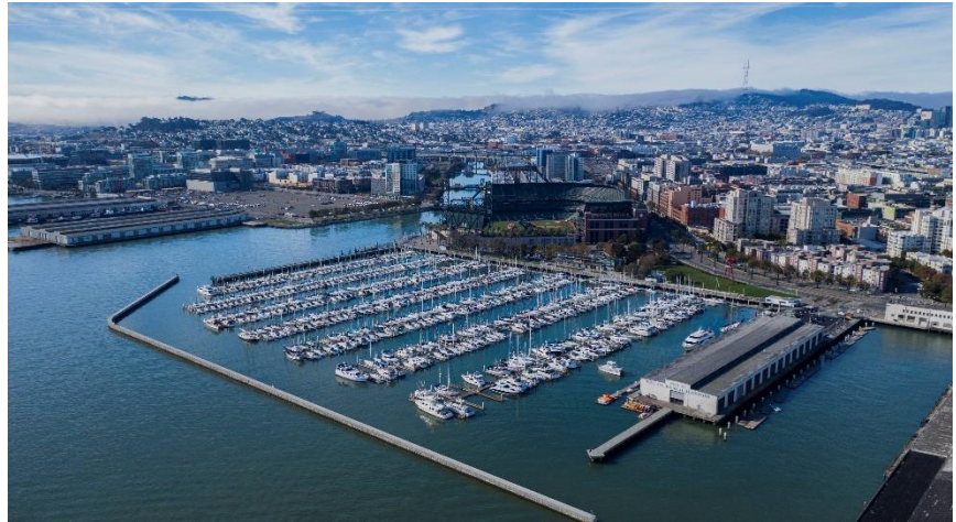
South Beach Harbor wave barrier ©Civic Edge Consulting
