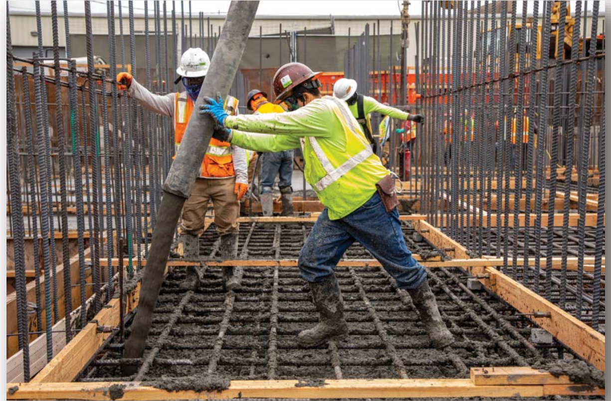
Power Distribution construction.
