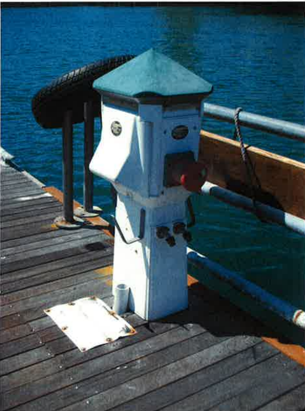
09-Electric Power Pedestal
