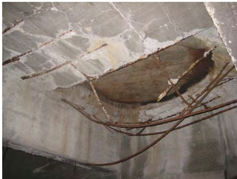
Figure 2 - Hole in Concrete Deck
