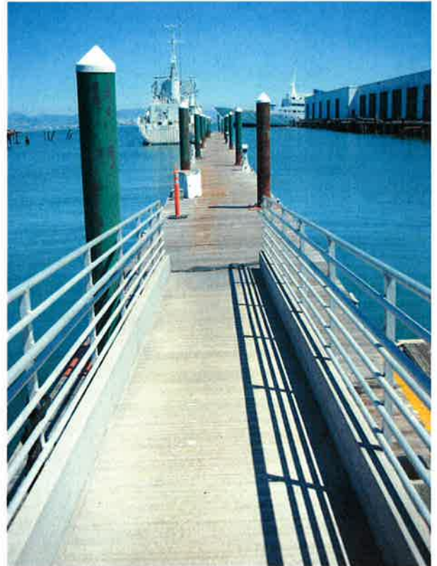
04-Access Ramp & Finger Pier
