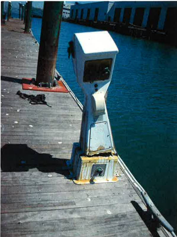
05B-Damaged Power Pedestal
