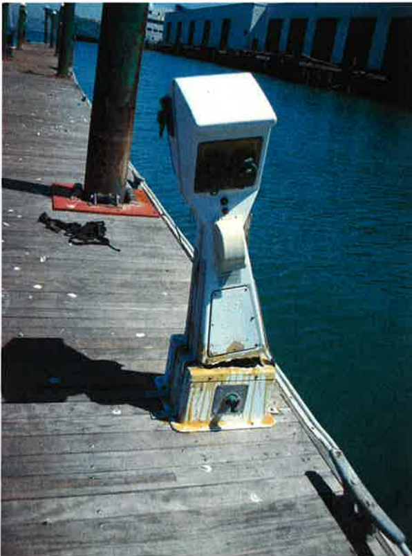
05B-Damaged Power Pedestal
