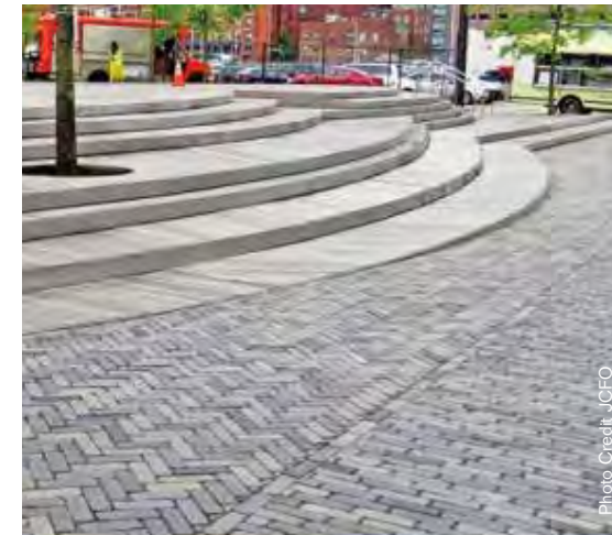
HARDSCAPE - PERMEABLE PAVING
