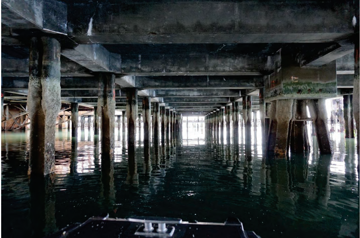
Figure 28 – Typical Condition of Piles , Beams & Deck
