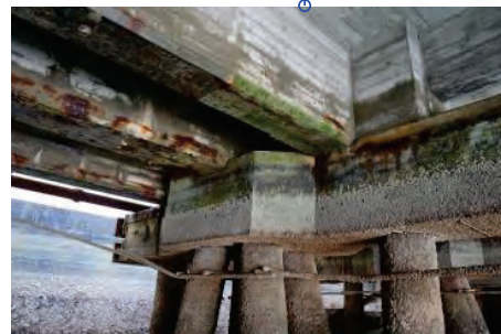
Typical Deck, Beam and Pile Cap condition
