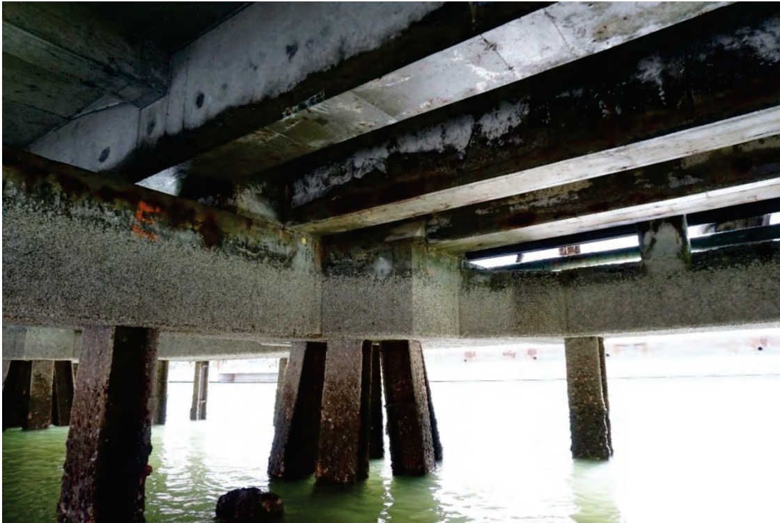
Figure 3 - Typical Condition Pile, Pile cap, Beam
