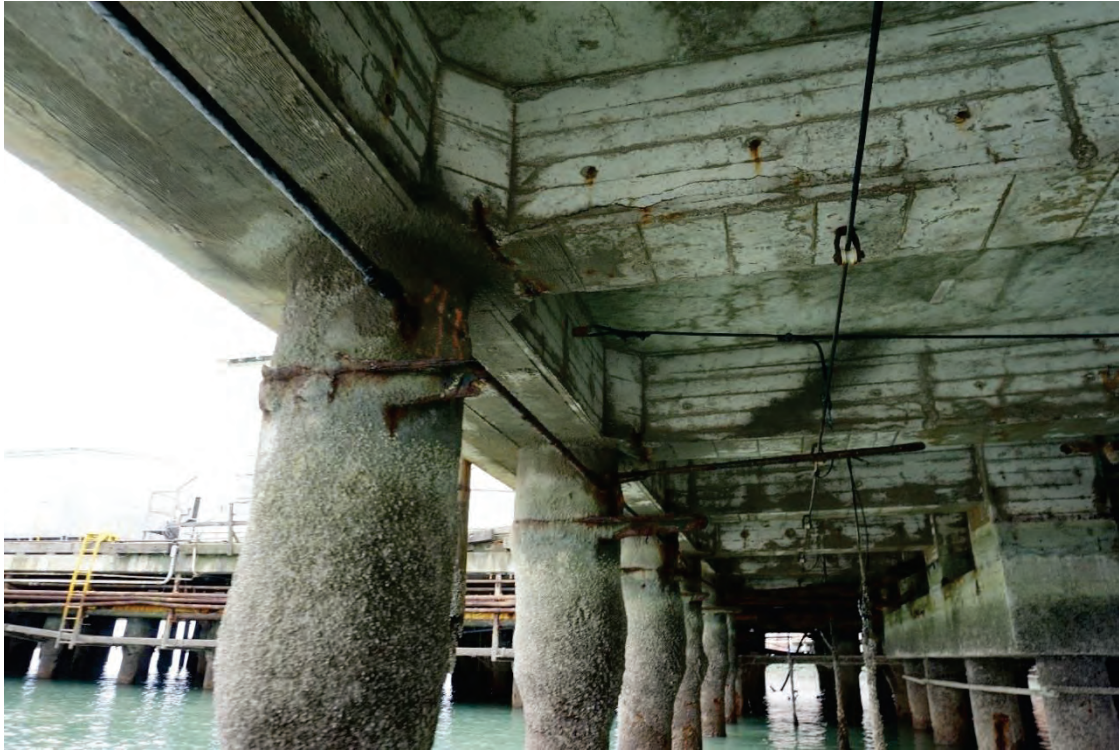
Figure 20 – Typical Beams and Pile Condition
