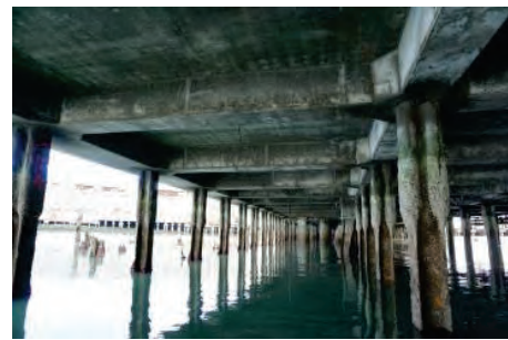
Typical Condition of Deck, Beam Pile
