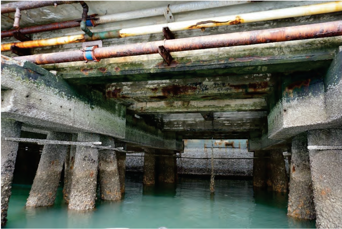
Figure 8 - Typical Conditions Beams, Piles, Pile caps
