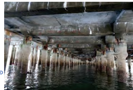
Typical Deck, Beam, Pile Cap Condition
