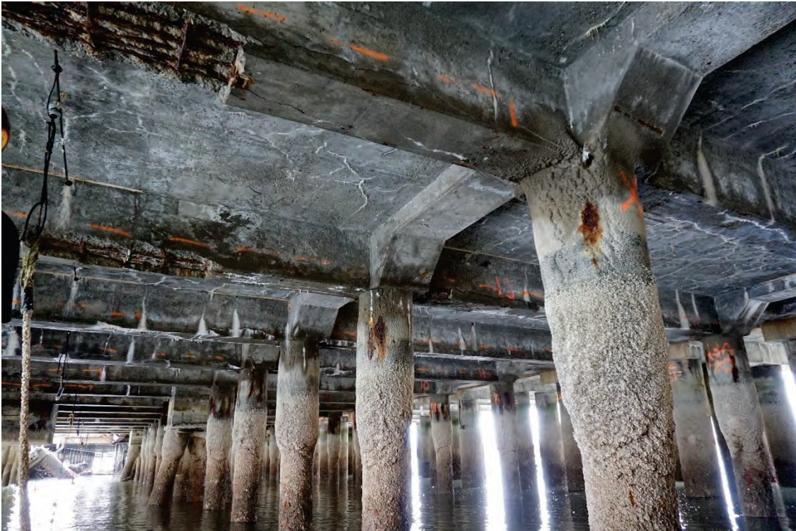
Figure 23 – Typical Condition of Piles, Pile Caps, Beams & Deck
