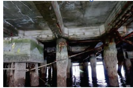
Beam, Pile Cap and Deck condition
