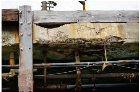
Spalled Deck
