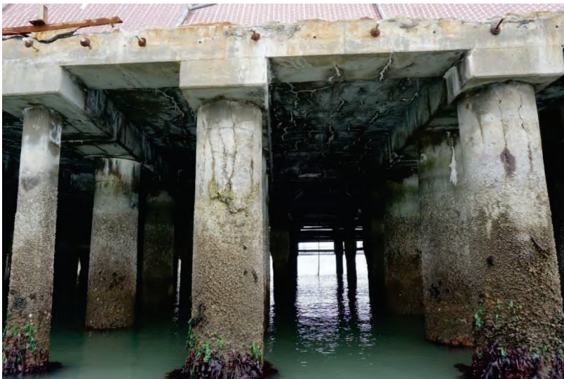
Figure 26 - Typical Pile and Deck Condition
