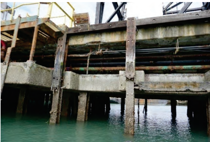
Figure 6 – Typical Deck Condition
