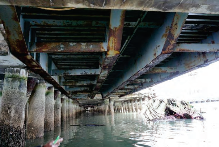
Figure 33 - Typical Condition of Steel Bridge Underside
