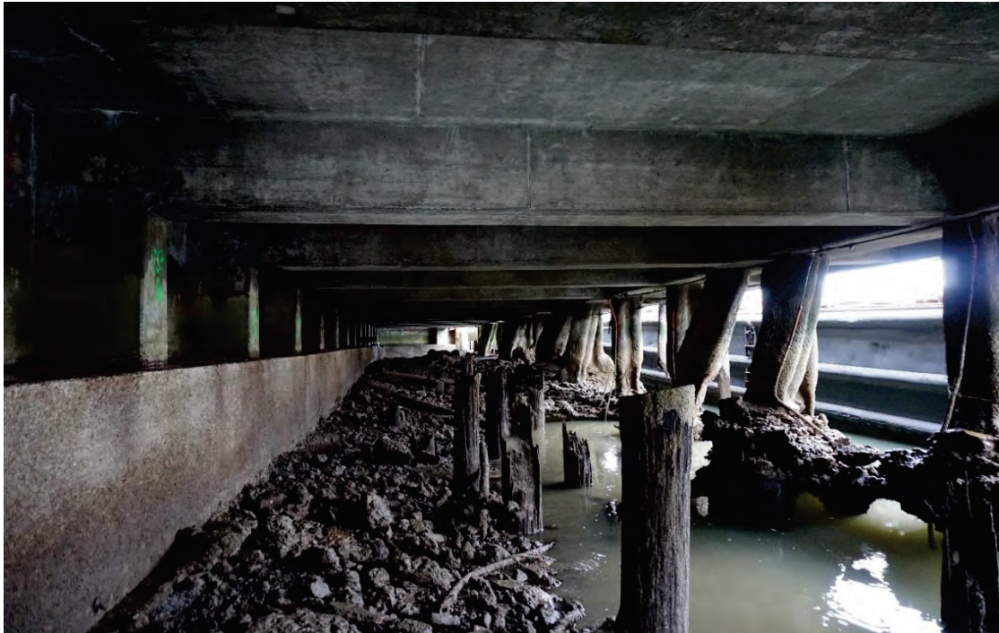
Figure 13 - Typical Condition of Beams and Piles
