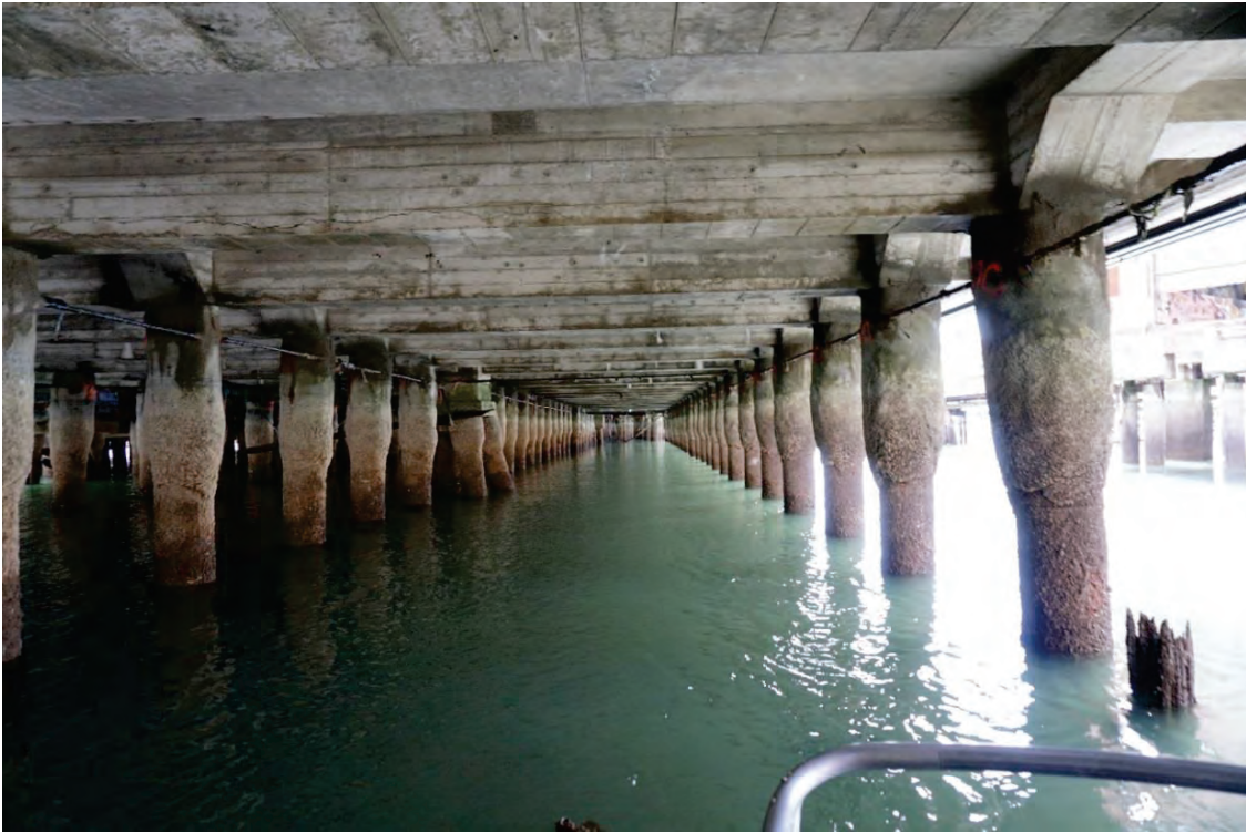
Figure 17 - Typical Condition of Beams and Piles
