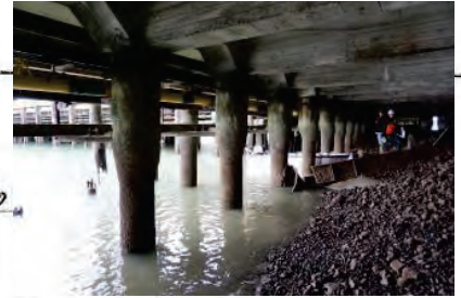
Typical Condition of Piles, Pile Caps, Decks
