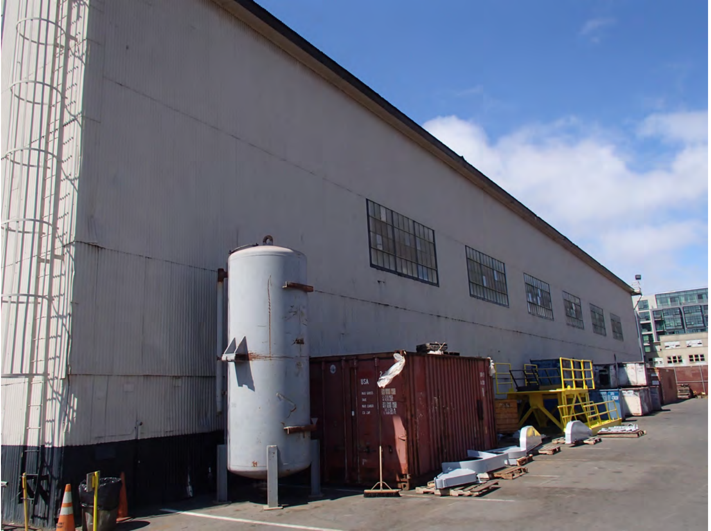
Photo 10. View of the north elevation
