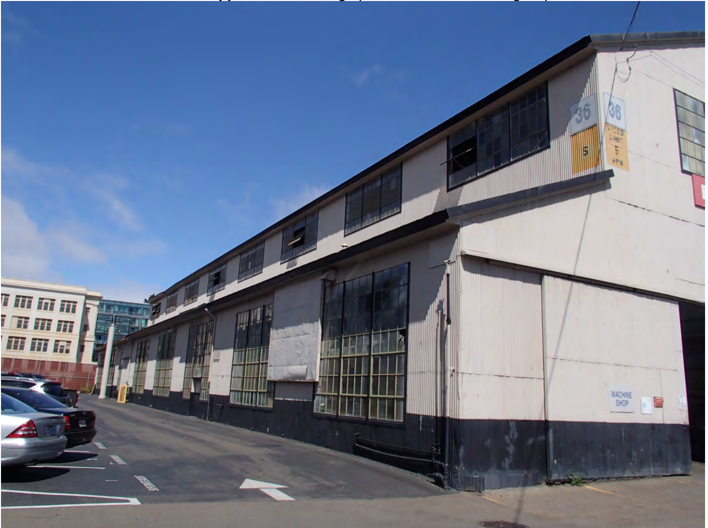
Photo 12. View of the south elevation
