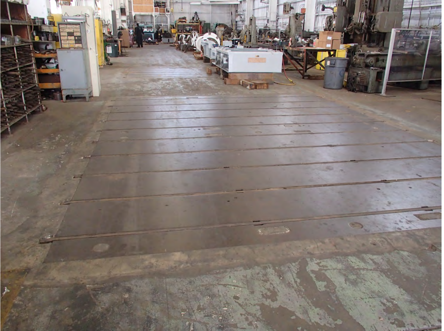
Photo 4. View of the interior floor slab
