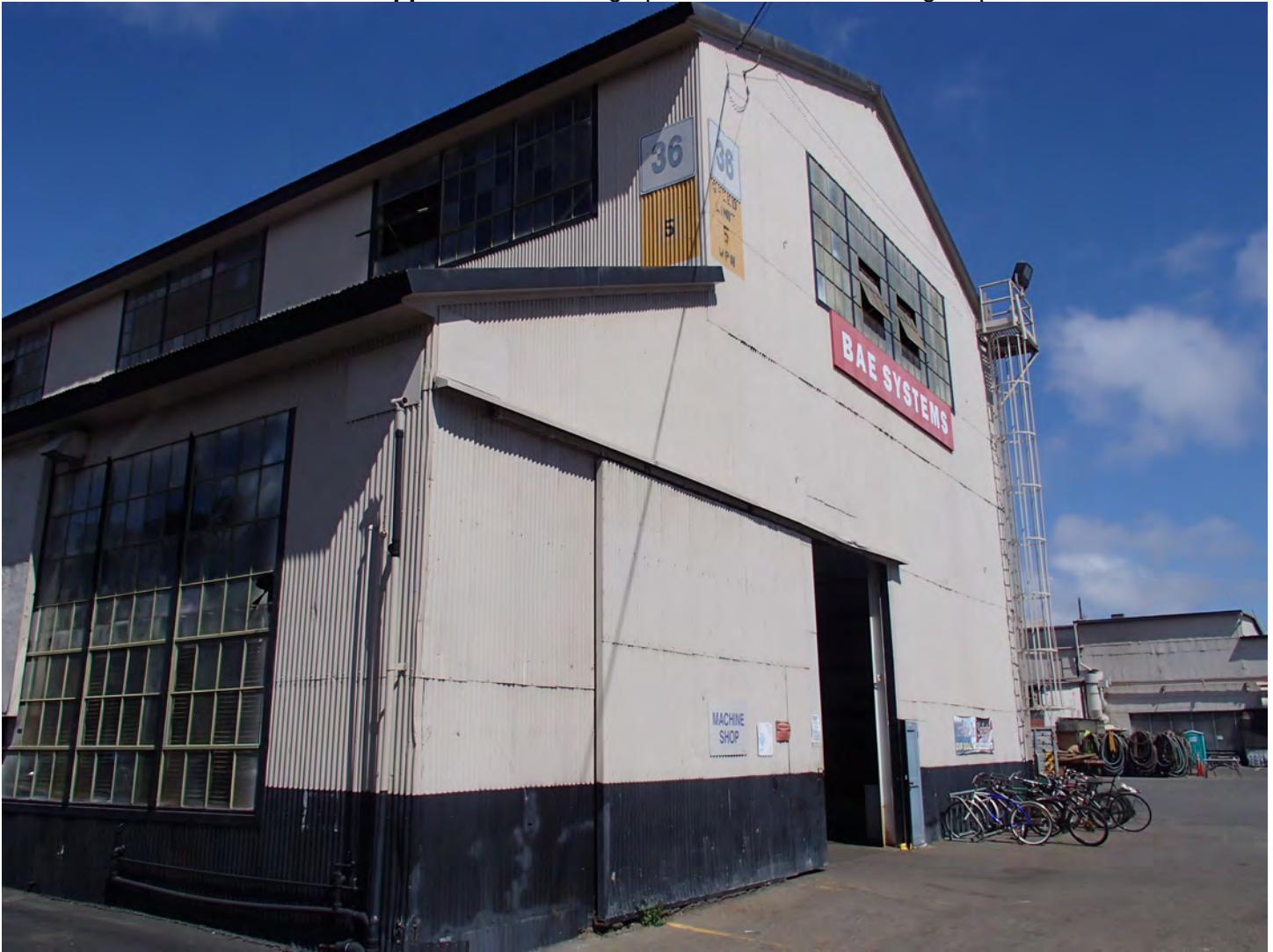
Photo 11. View of the east elevation
