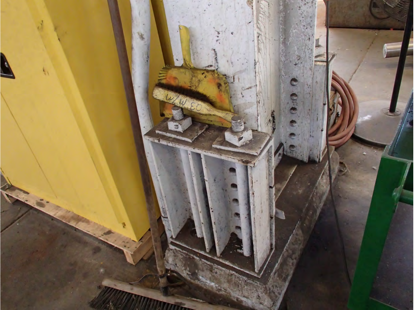
Photo 3. View of the interior steel column base connection
