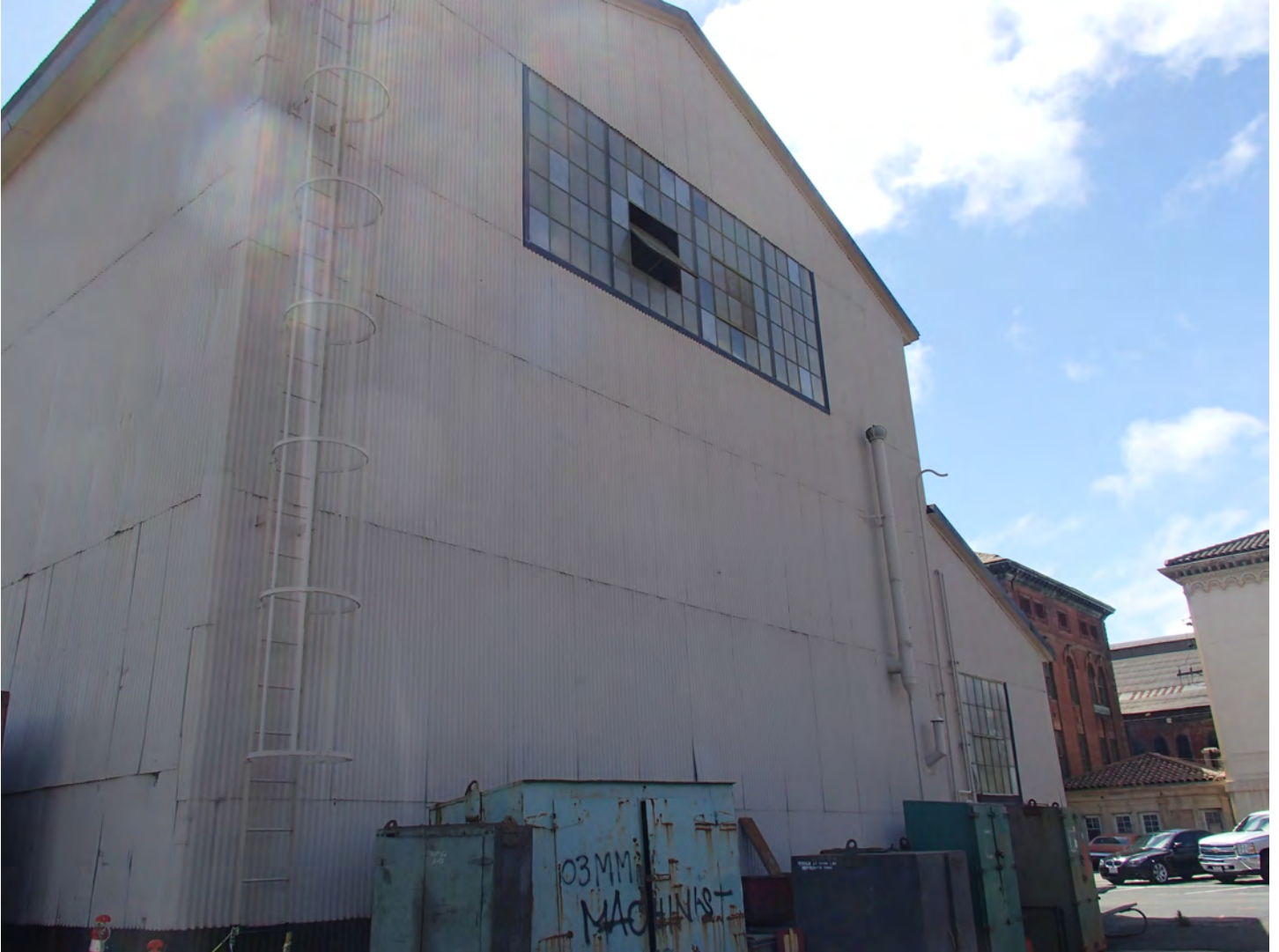
Photo 8. View of the west elevation
