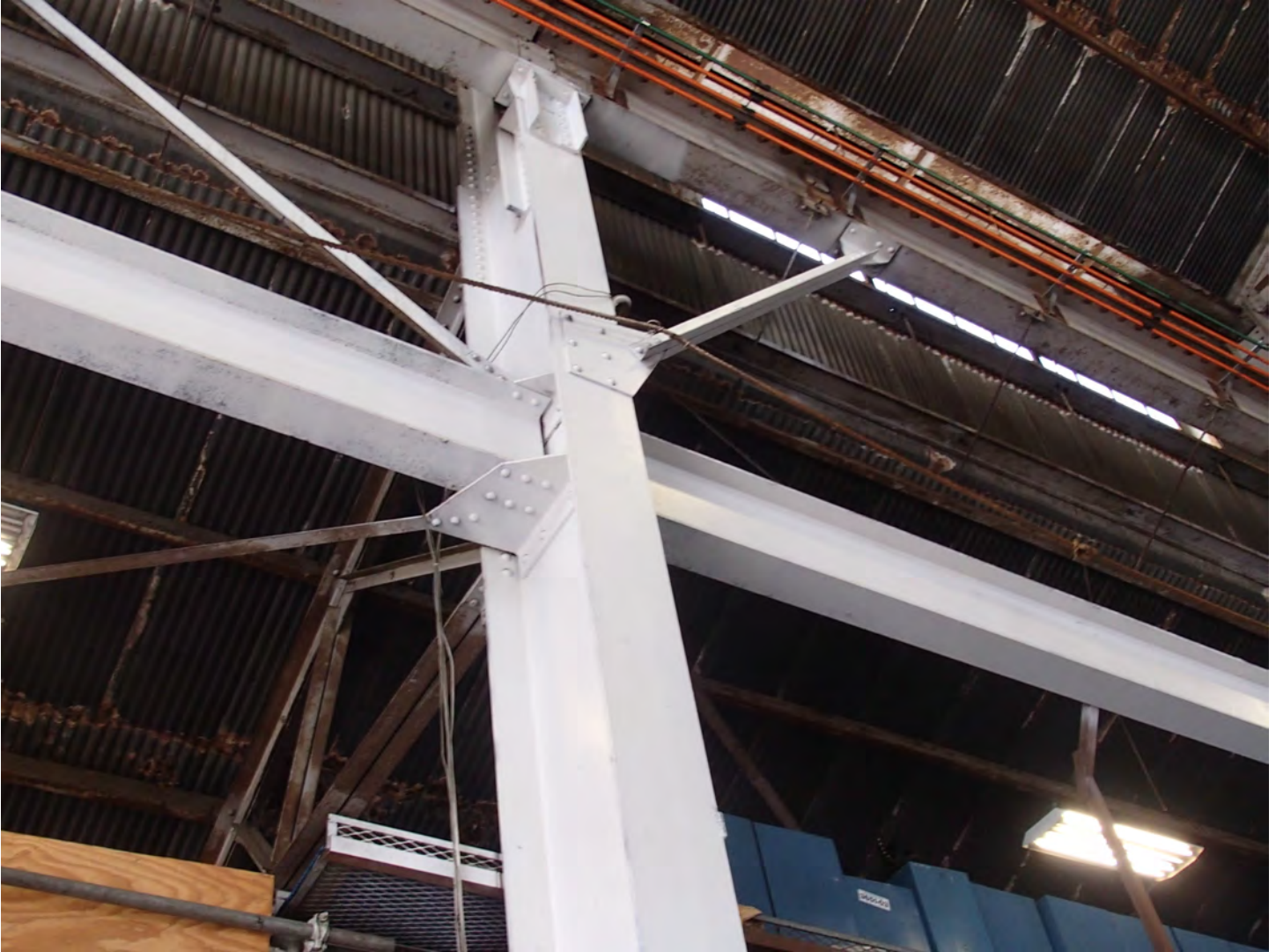
Photo 6. View of the interior steel column
