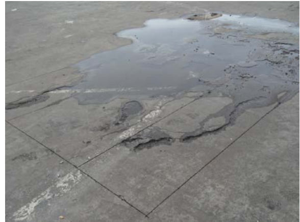
Saw cutting and concrete replacement
