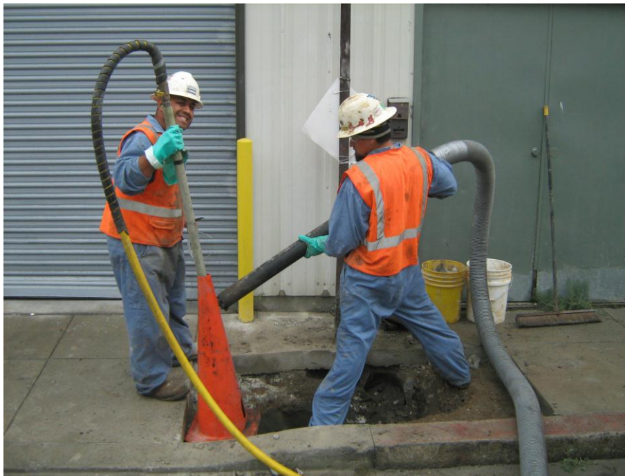
Photograph 5 – Air-knifing in sidewalk at suspect vent pipe at Building 49
