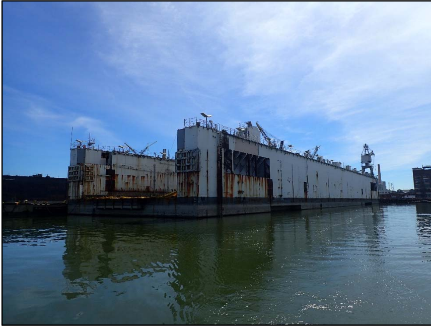
Photograph 1 : Overall view of Dry Dock EUREKA, looking southeast.
