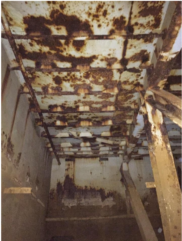
13. Roof stiffeners at Tank 6A
