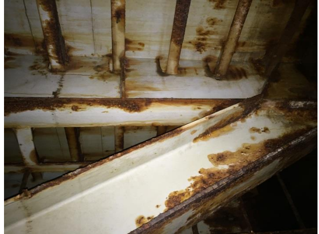
16. Roof stiffeners and braced frame at Tank 20A
