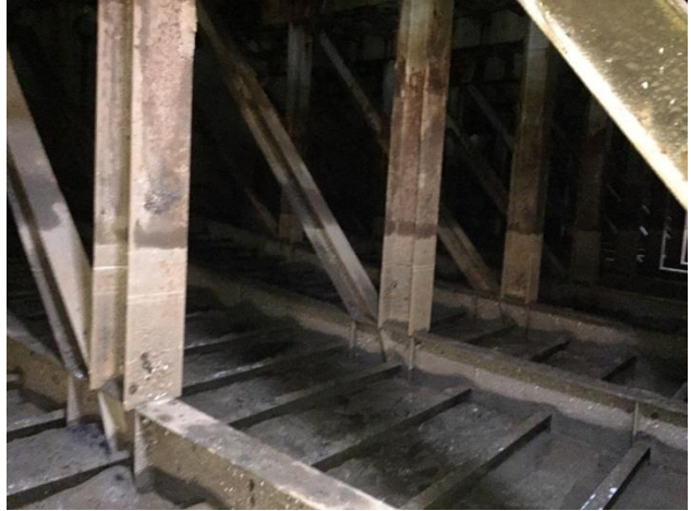
12. Braced frames at Tank 9
