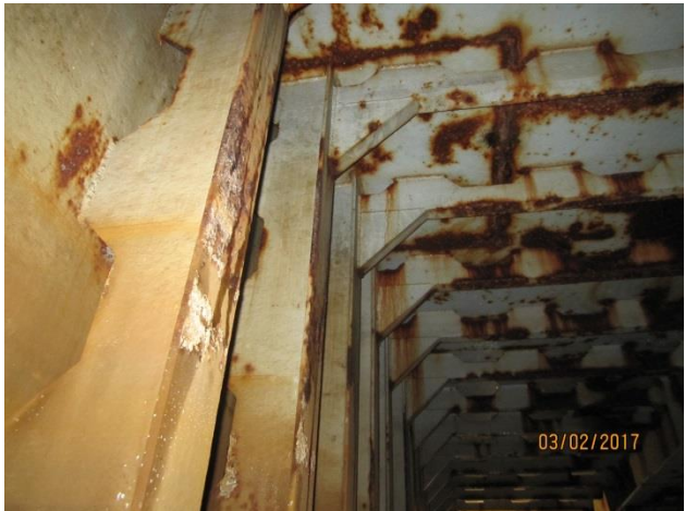
21. Wall stiffeners at Tank 6
