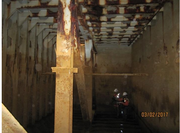
20. Roof stiffeners and braced frame at Tank 6
