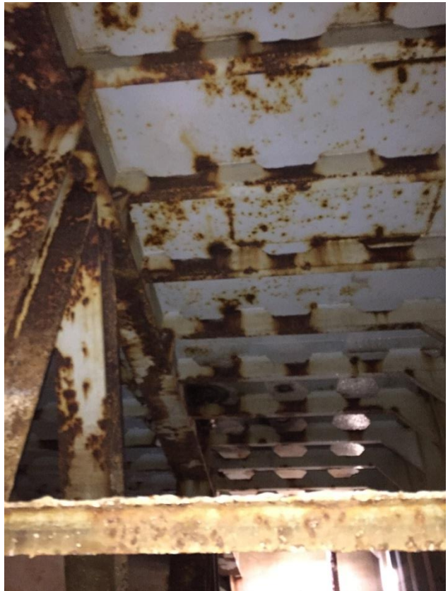
14. Roof stiffeners at Tank 6A
