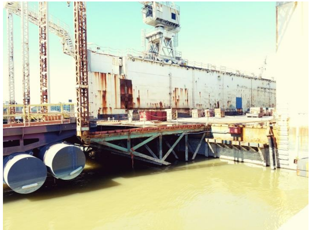
4. Ramp at south end
