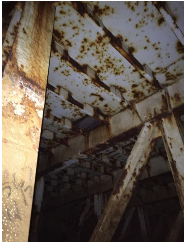
18. Roof stiffeners and braced frame at Tank 5
