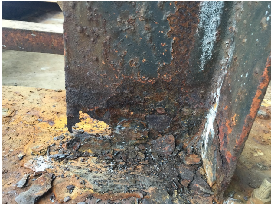
Figure 20 – Deteriorated base connection at corner column.
