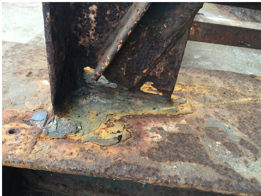
Figure 17 – Deteriorated base connection at braced column.
