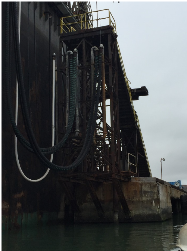
Figure 11 – Full view of stair tower framing.
