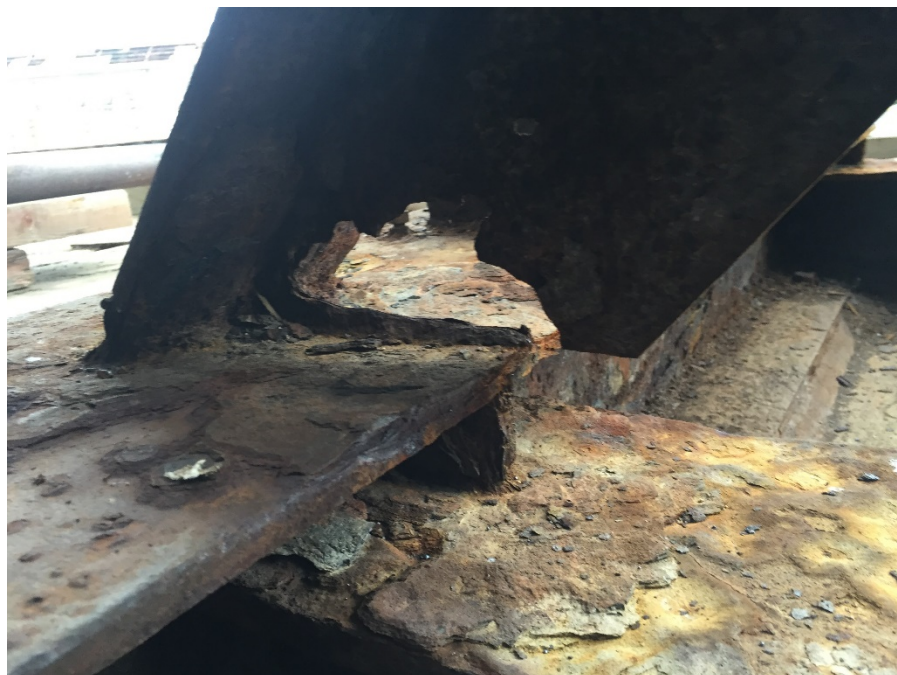
Figure 18 – Complete loss of cross section at angled brace support.
