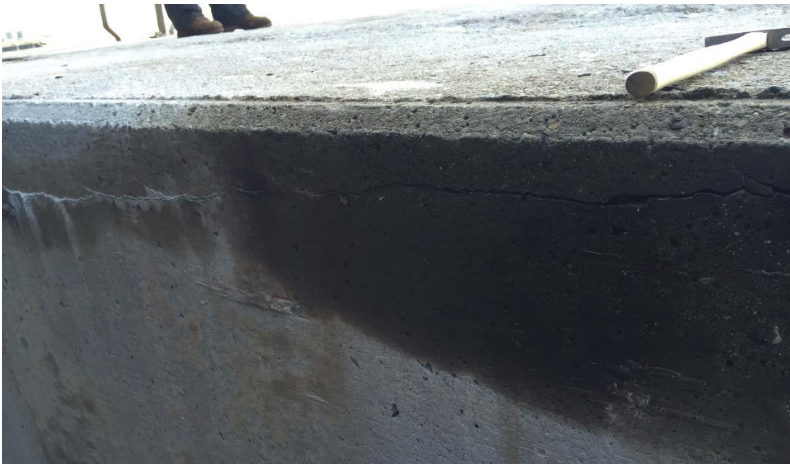
Figure 8 – Close-up view of horizontal crack near top corner of dolphin deck structure (D4).
