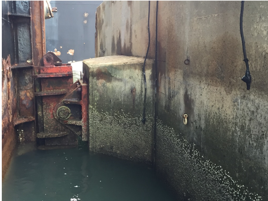
Figure 1 – General view of dry dock gripper assembly mounted at concrete extension at face of concrete dolphin (D4).
