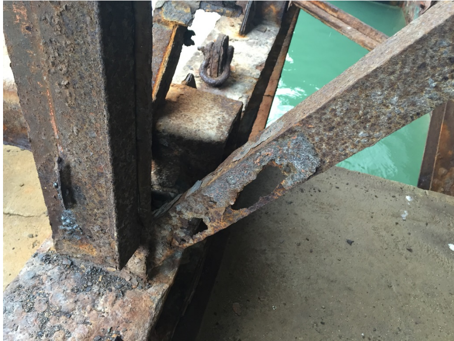
Figure 19 – Complete loss of section at diagonal brace.
