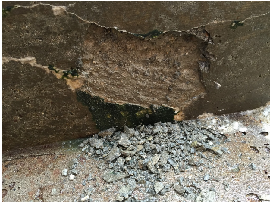
Figure 6 – Close-up view of spalling and soft concrete observed at east face of dolphin (D2).
