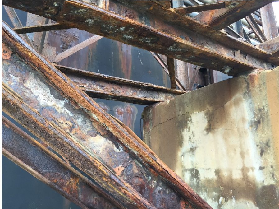
Figure 25 – Heavily corroded base horizontal beams and diagonal struts. Approximately 50% to 60% of original cross section remains.
