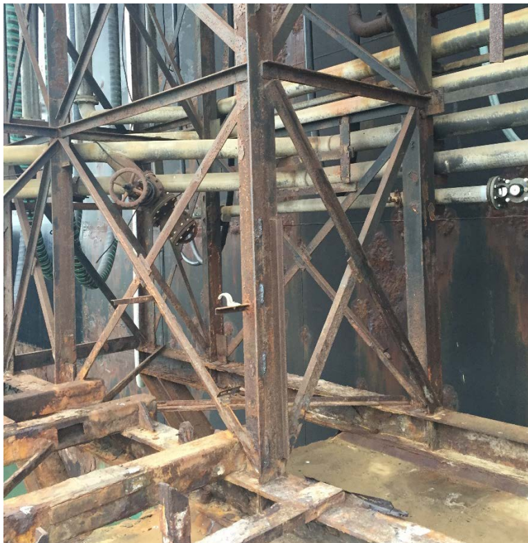
Figure 13 – View of heavily corroded base region of steel frame.
