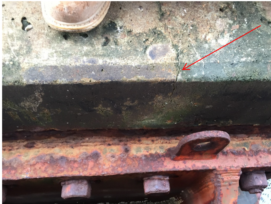
Figure 4 - View of typical crack in concrete extending from gripper plate at dolphin (D3).
