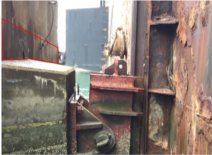
Figure 5 – Location of concrete spalls at east face of dolphin (D2).
