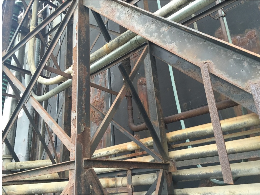
Figure 15 – View of upper portions of steel frame in good condition.
