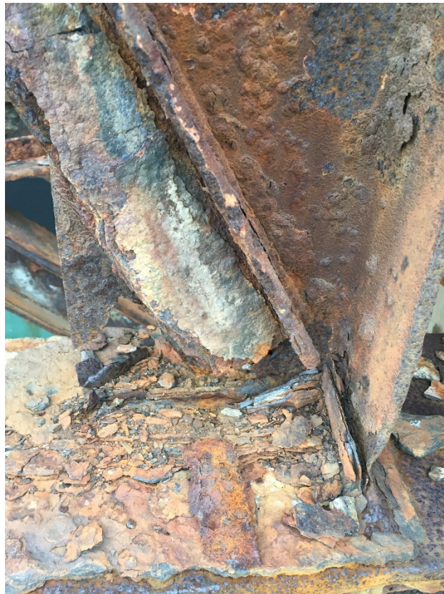
Figure 22 - Heavily scaled connection at braced column connection.
