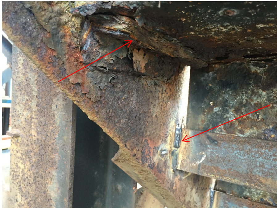
Figure 24 – View of deterioration at shear tab support between stringer and stair tread (upper). Repaired stair tread connection (bottom right).
