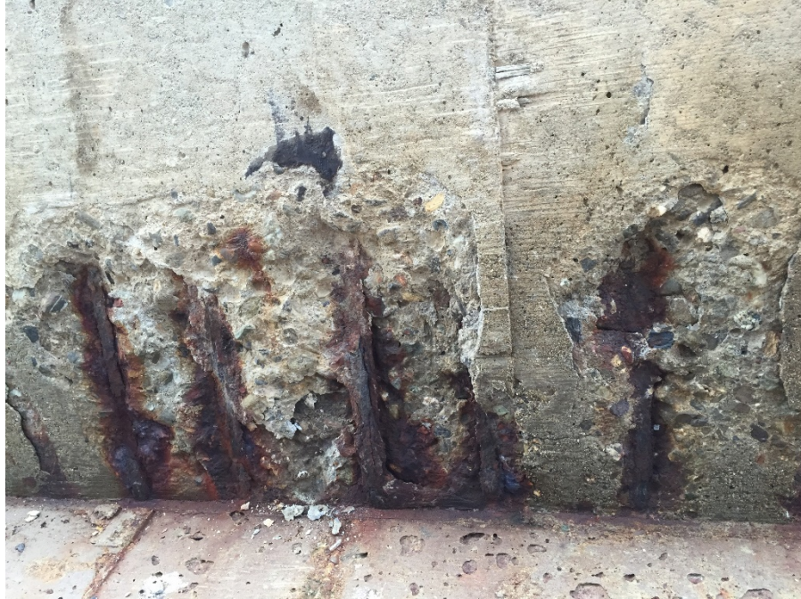
Figure 7 – Close-up view of open corrosion spall at east face of dolphin (D3). Note exposed steel reinforcing.
