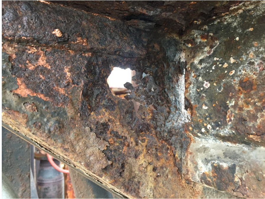
Figure 23 – Complete loss of cross section at web of stair stringer.
