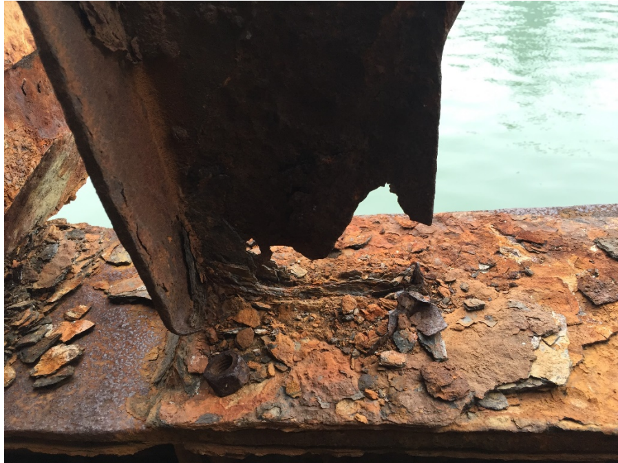
Figure 21- Complete loss of cross section due to corrosion at corner column base connection.
