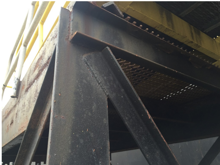
Figure 16 – Upper region of tower frame in excellent condition. Paint coating remains in good condition.
