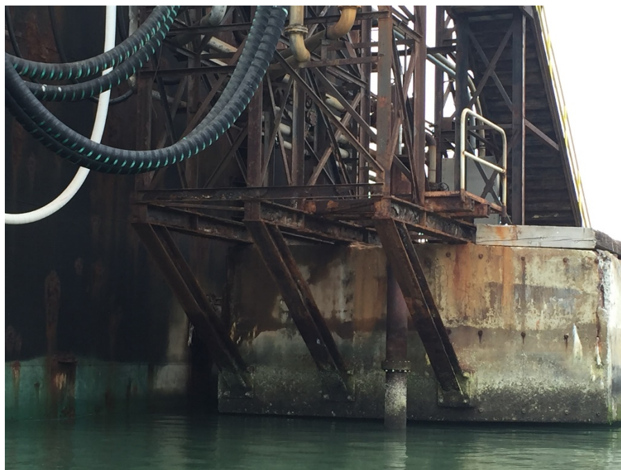
Figure 12 – View of lower frame and support framing at dolphin D1.
