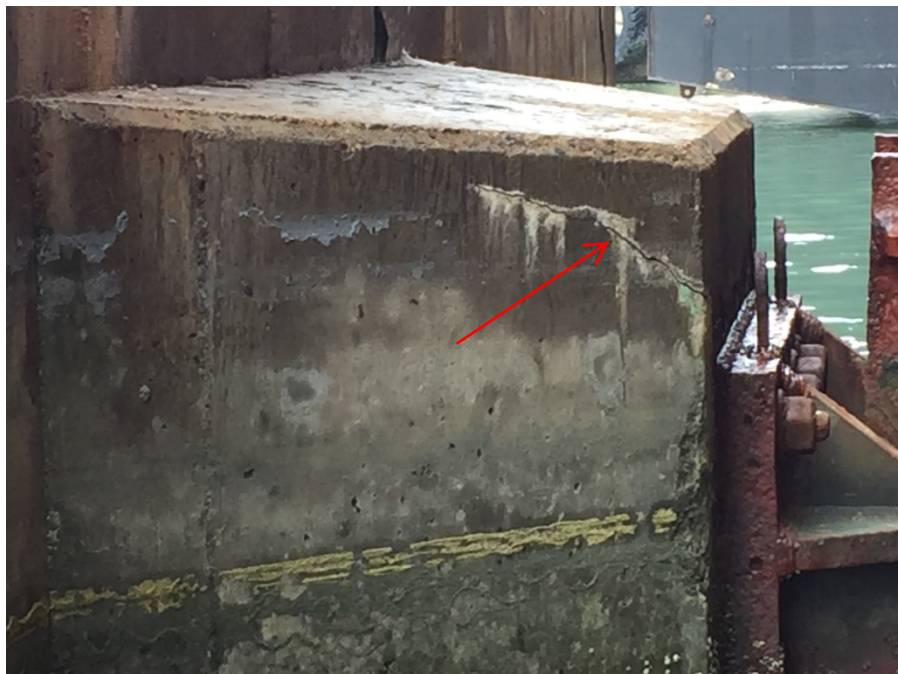
Figure 2 – Close-up view of crack extending from top corner of gripper plate to side face and upwards at dolphin (D2).
