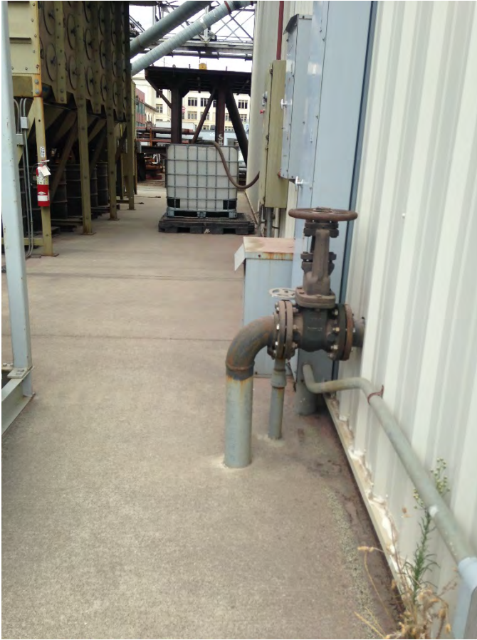
Figure 24. Compressed air 4" service valve size
