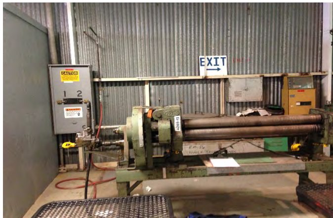
Figure 20. Compressed air 6" service size valve
