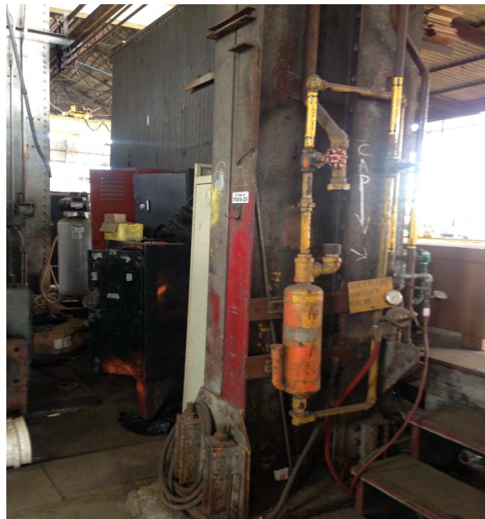
Figure 48. Oxygen/Acetylene Welding gas service size is 2"
