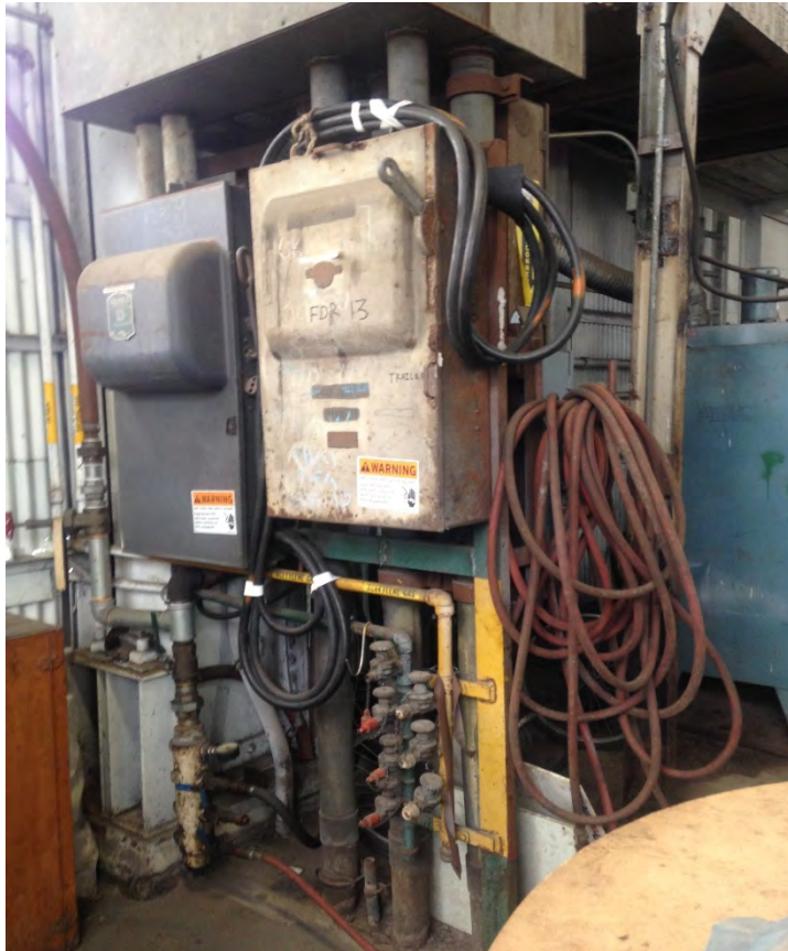
Figure 9. Compressed air and natural gas distribution
