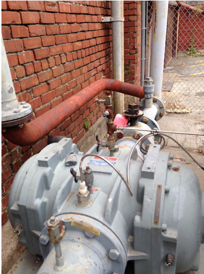
Figure 29. PG&E gas meter 245G-40, primary gas service to the Shipyard
