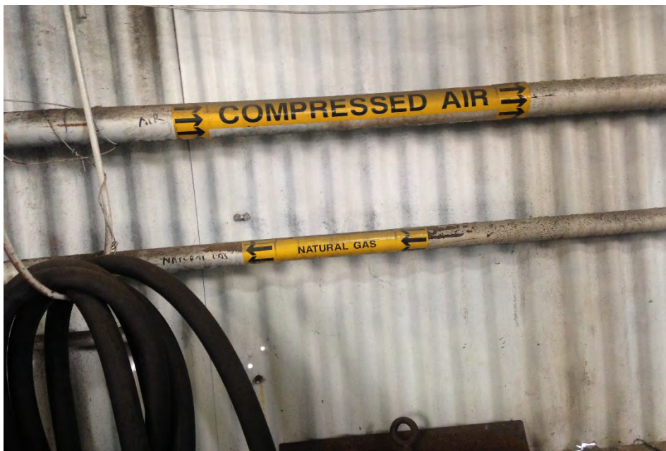
Figure 32. Natural gas 1.5" service size
