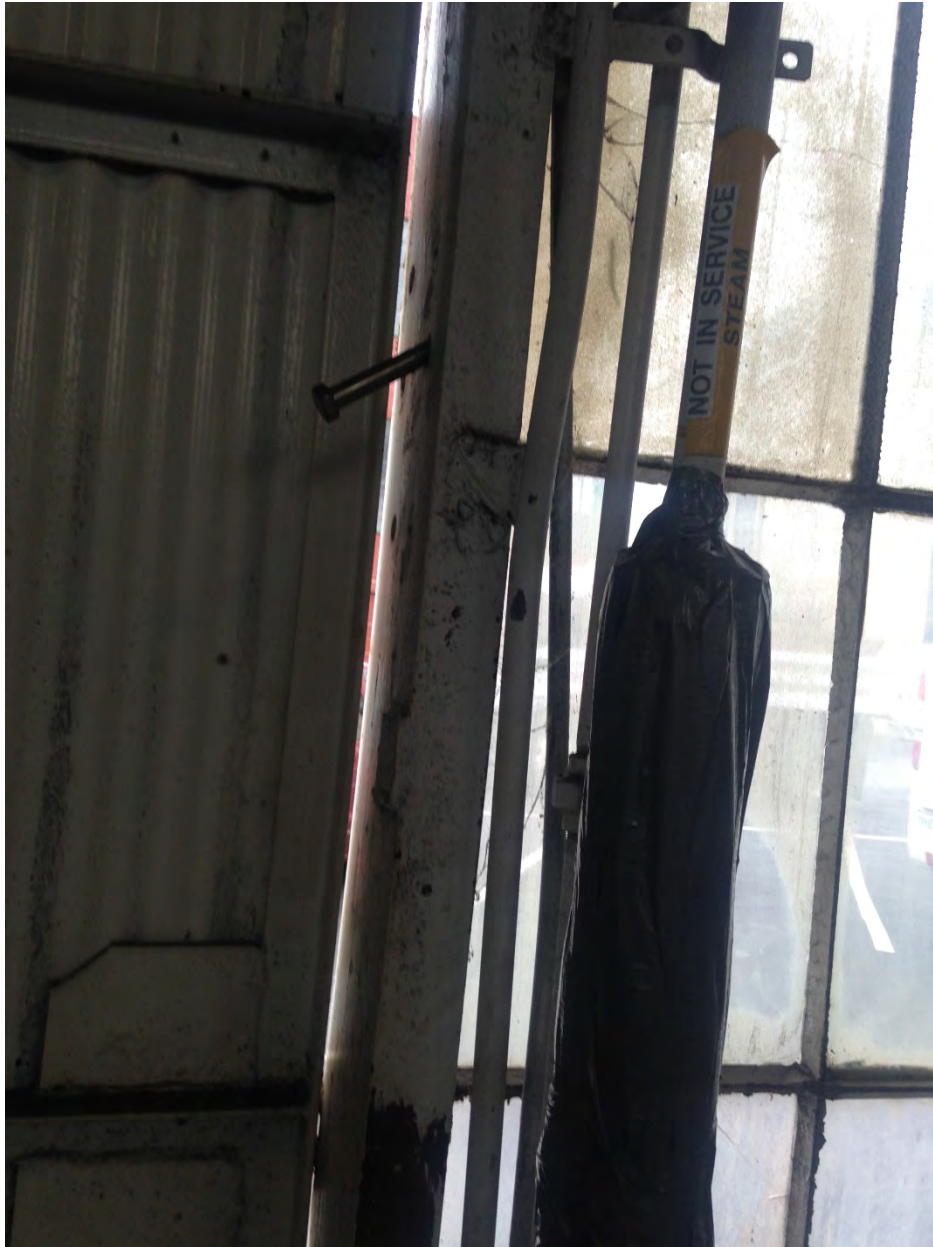
Figure 28. Steam service 1.5" service size
