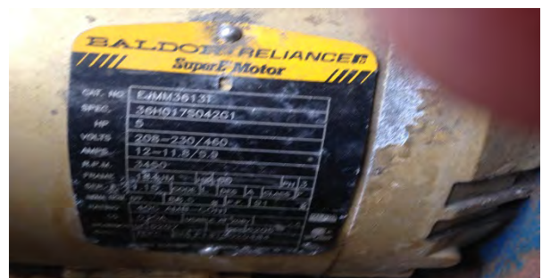
Figure 5. Cooling Tower Pump Nameplate
