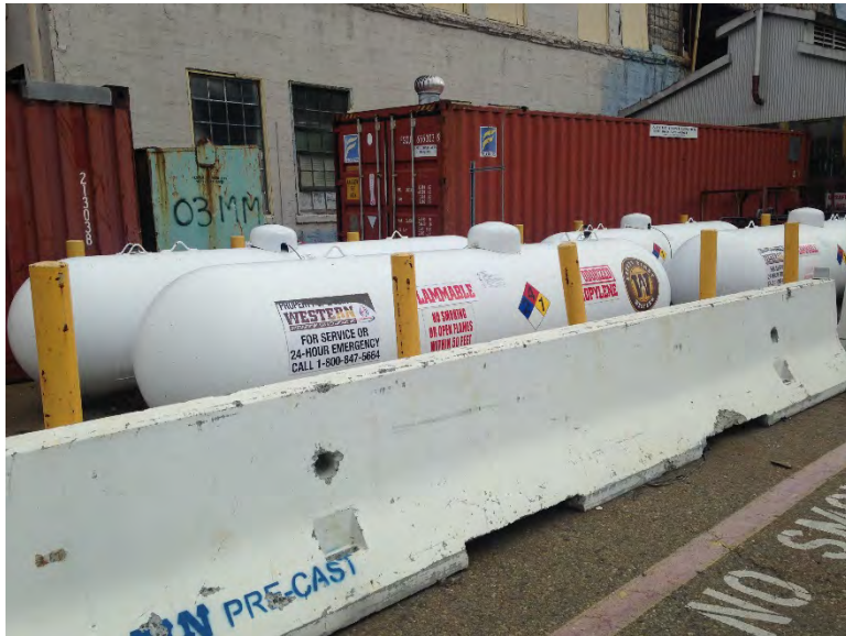
Figure 44. Propylene tanks
