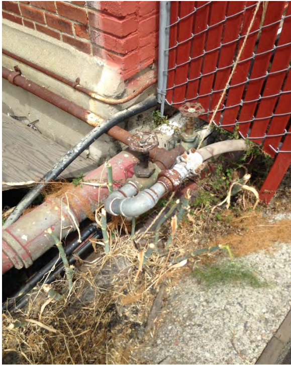
Figure 22. Compressed air 2" service size
