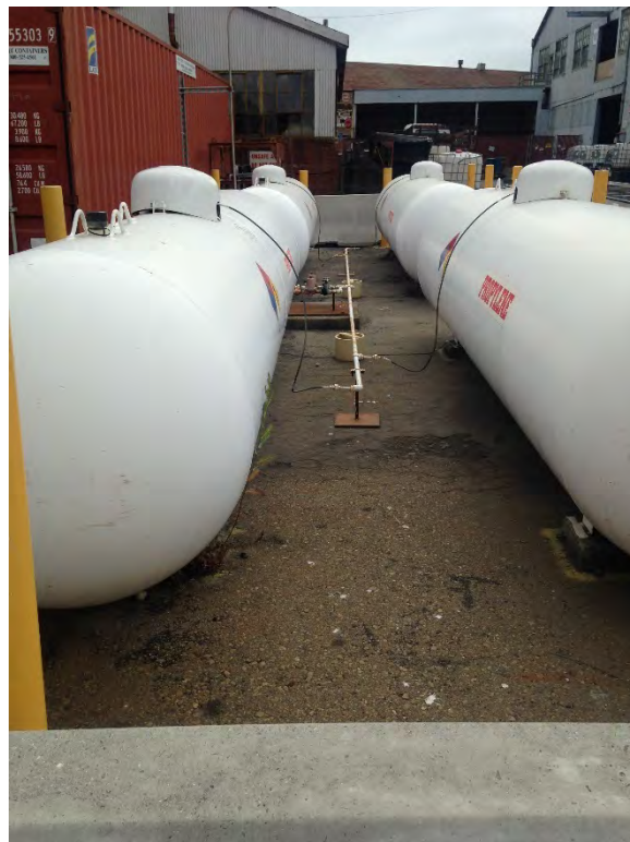
Figure 45. Propylene tanks
