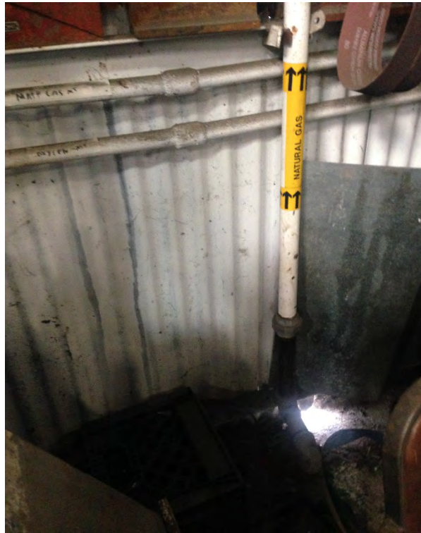
Figure 31. Natural gas 1.5" service size
