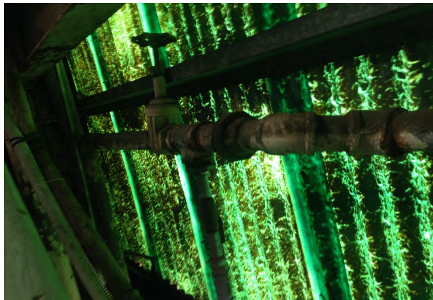
Figure 17. 2" compressed air service valve located on 2 nd floor adjacent to stairs
