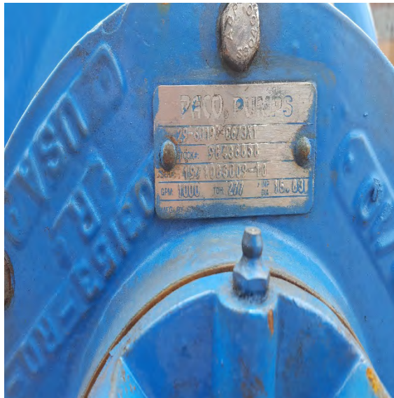
Figure 52. 75 HP Fresh Water Booster Pump nameplate (2 pictures)
