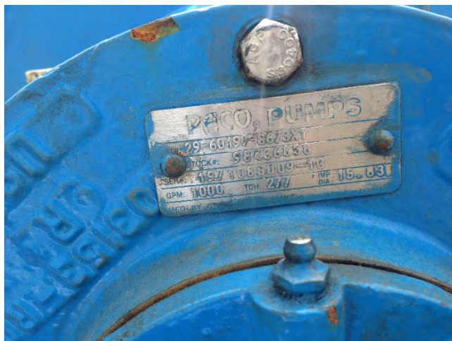
Figure 54. 250 HP Pier 3 Salt Water Pump (P3SWP) nameplates (2 pictures)
